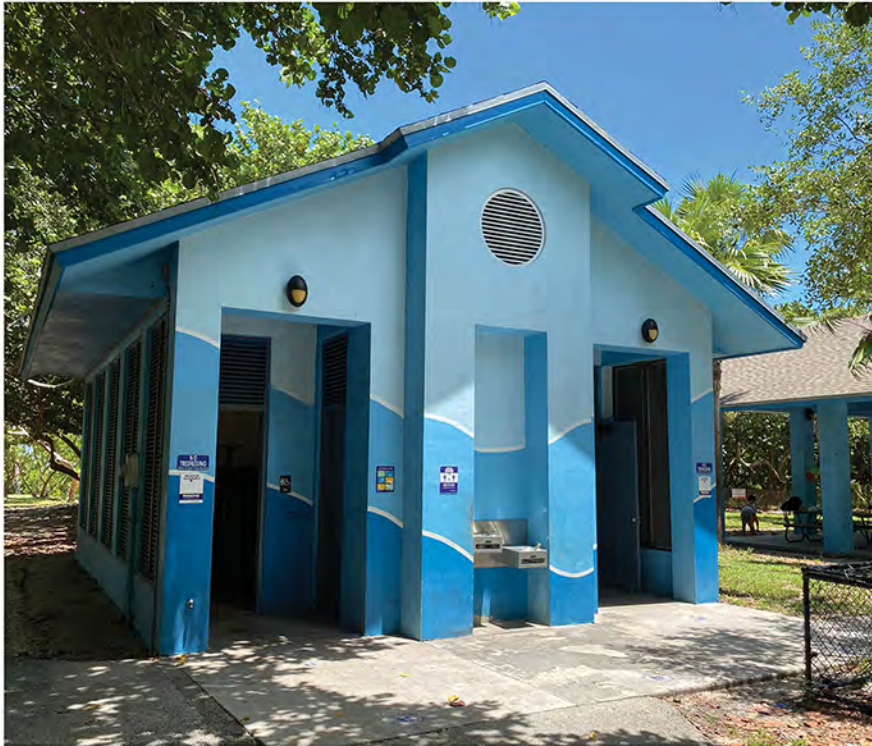
Existing Conditions - Exterior
