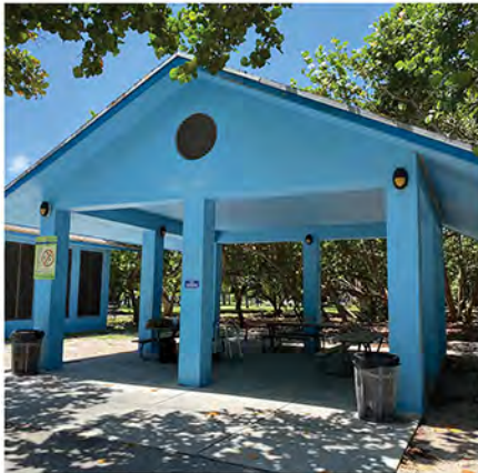
Concrete Shelters - Existing Conditions
