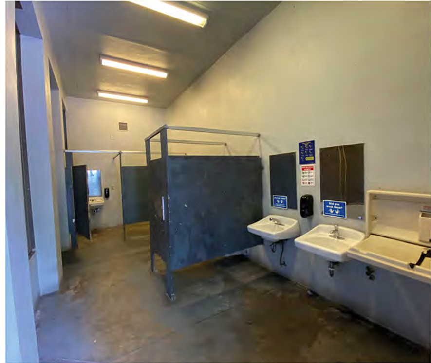
Existing Conditions - Interior
