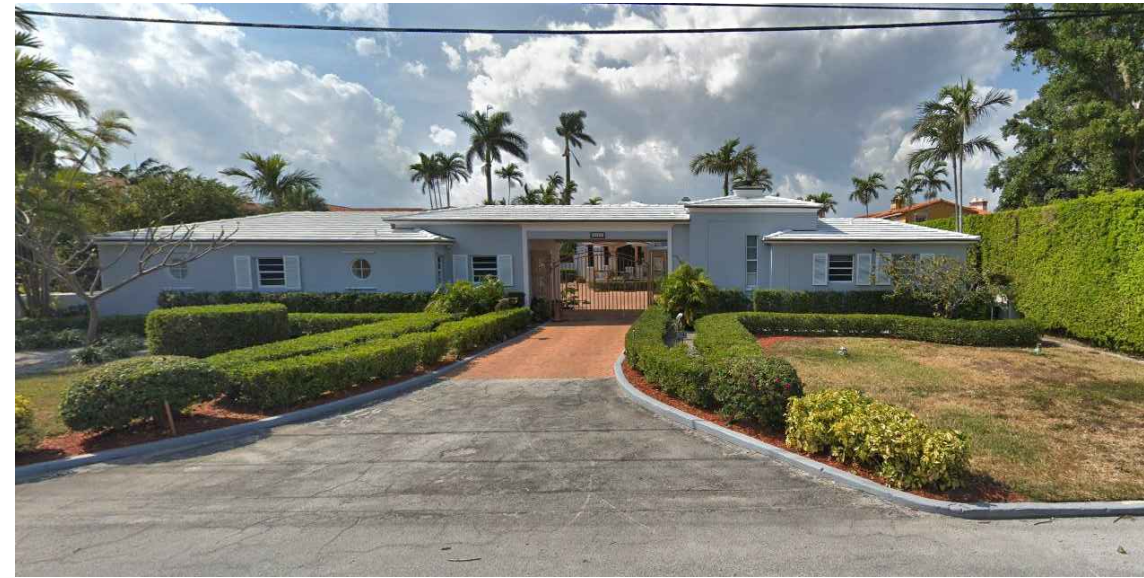
2. 6324 NORTH BAY ROAD
