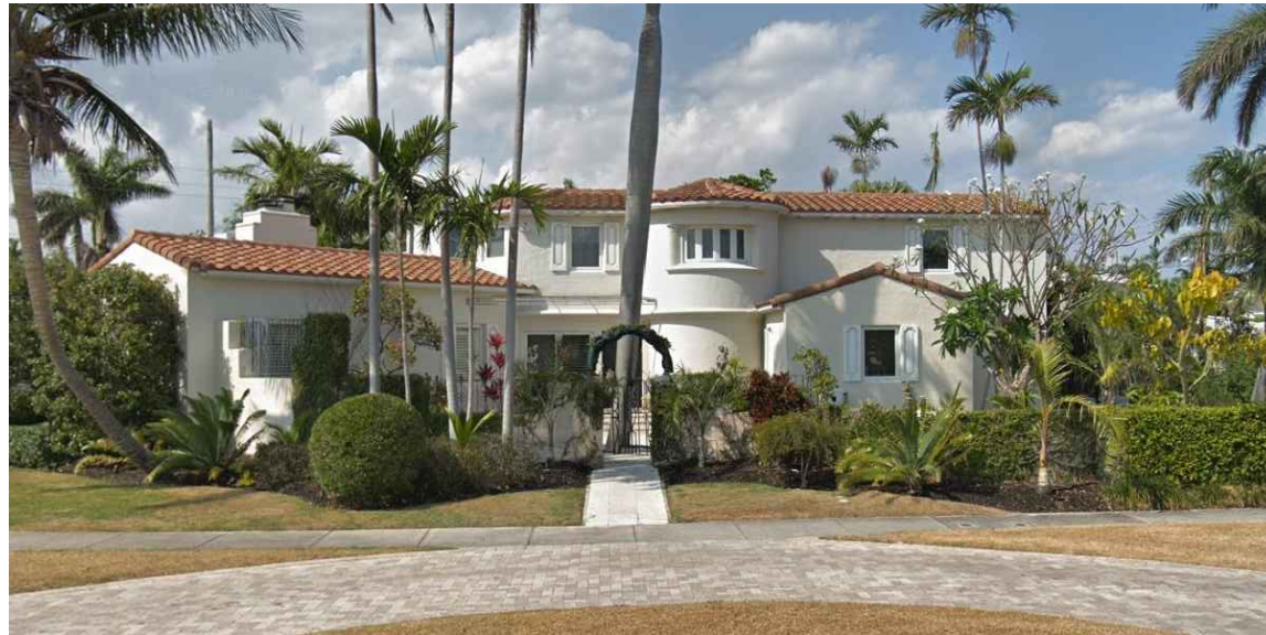
1. 6361 NORTH BAY ROAD
