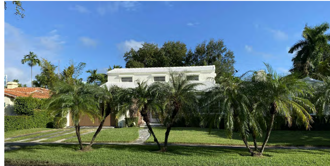
2. 6371 NORTH BAY ROAD
