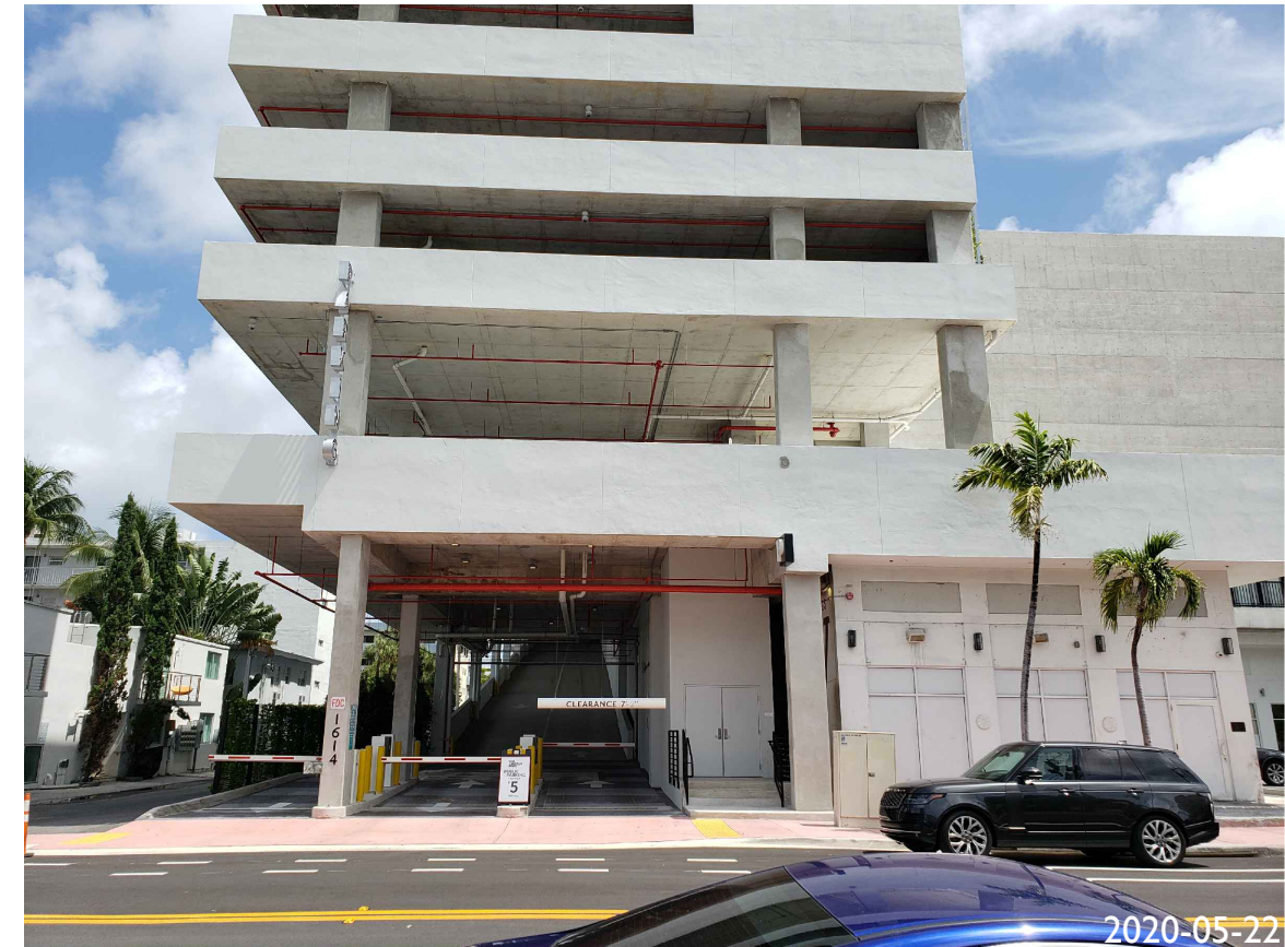
6. 1212 LINCOLN ROAD BUILDING - ENTRANCE TO GARAGE
