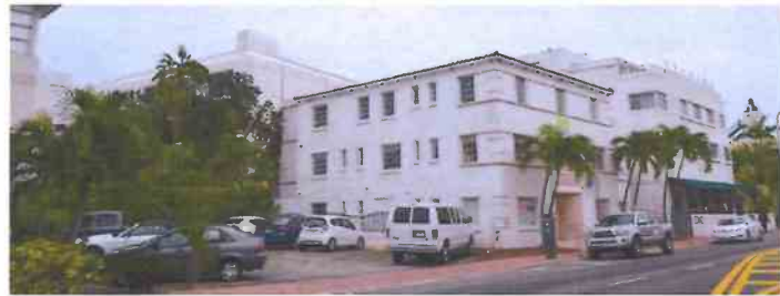
President Villa Hotel 1425 Collins Av, ground level addition
