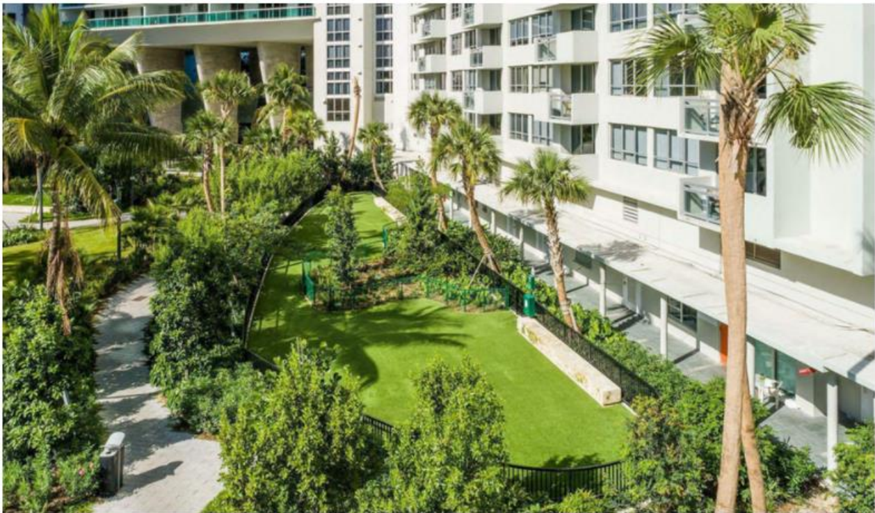
WORK COMPLETED: PHOTO OF SOUTH DOG RUN
