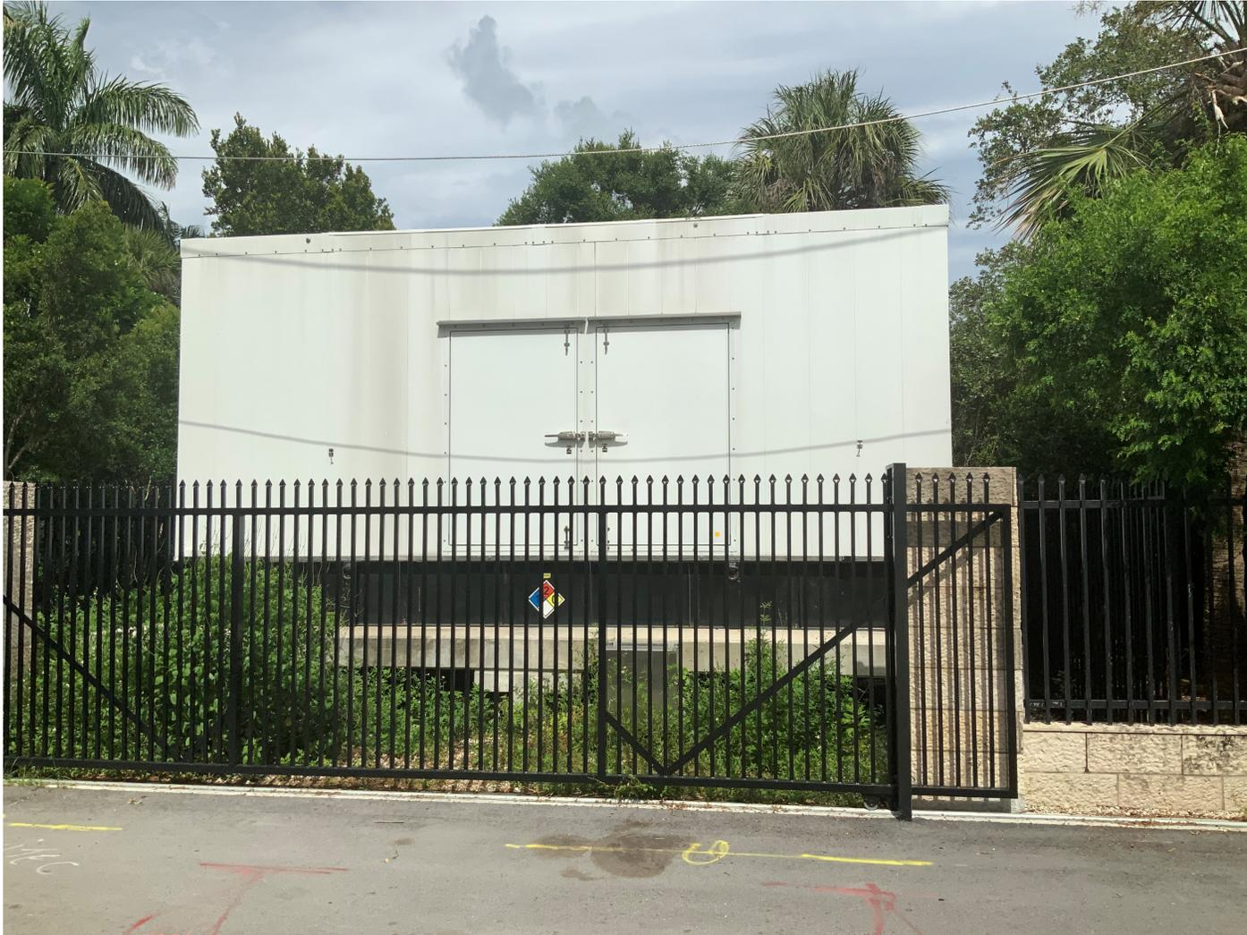
The **emergency generator** will power the entire Storm Water treatment system if there is a loss of power.
