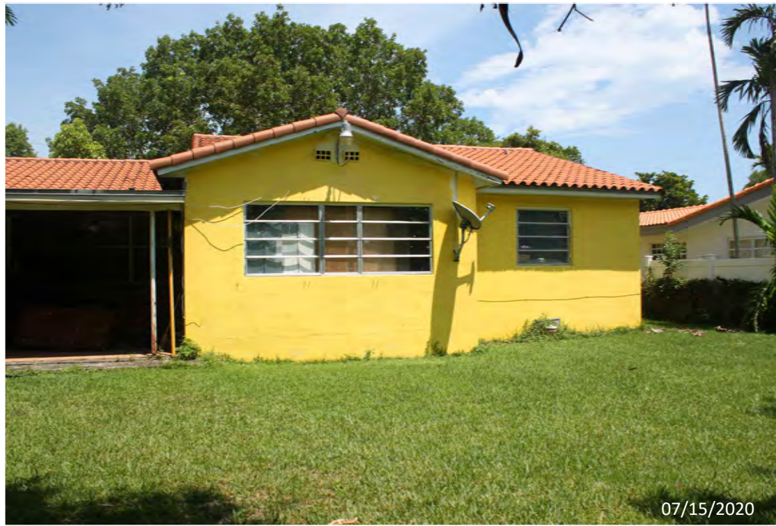
2. REAR EXISTING HOME
