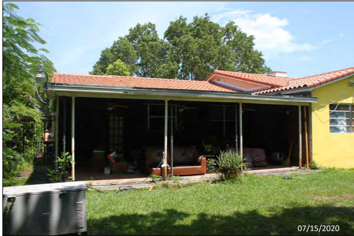
1. REAR EXISTING HOME NORTH WEST CORNER
