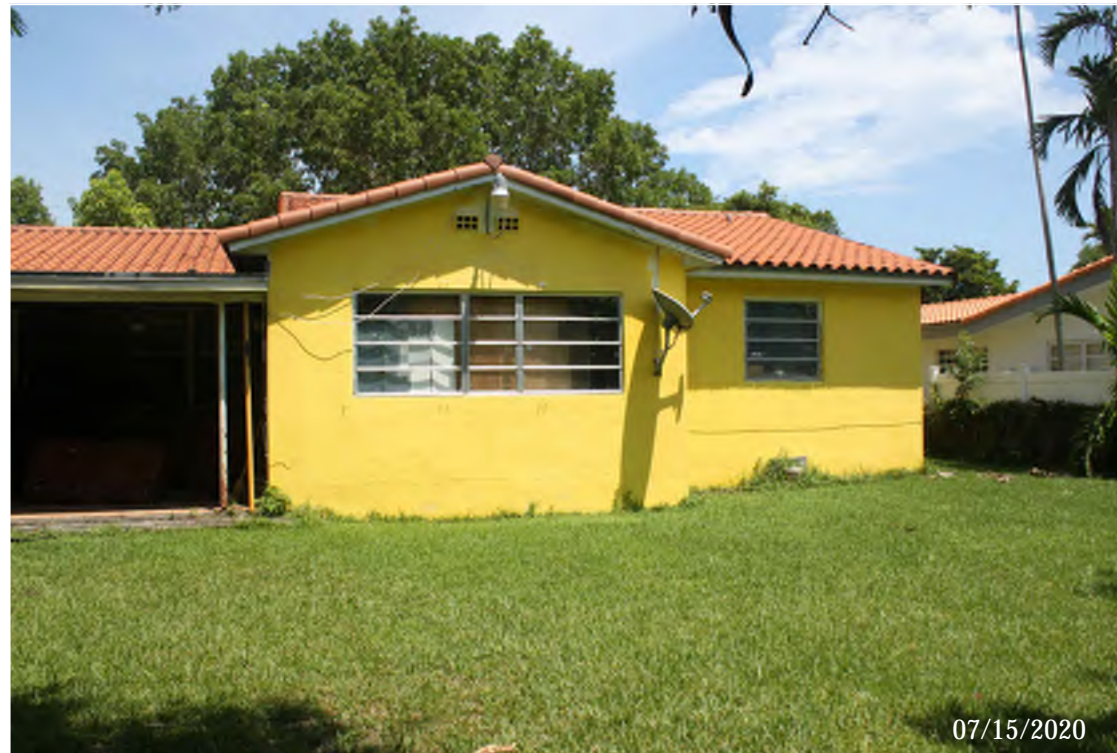
2. REAR EXISTING HOME
