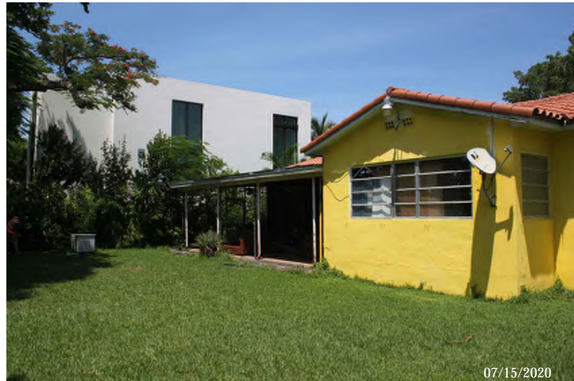
3. REAR EXISTING HOME SOUTH WEST CORNER
