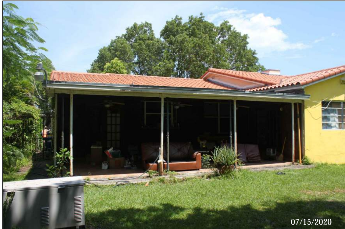
1. REAR EXISTING HOME NORTH WEST CORNER
