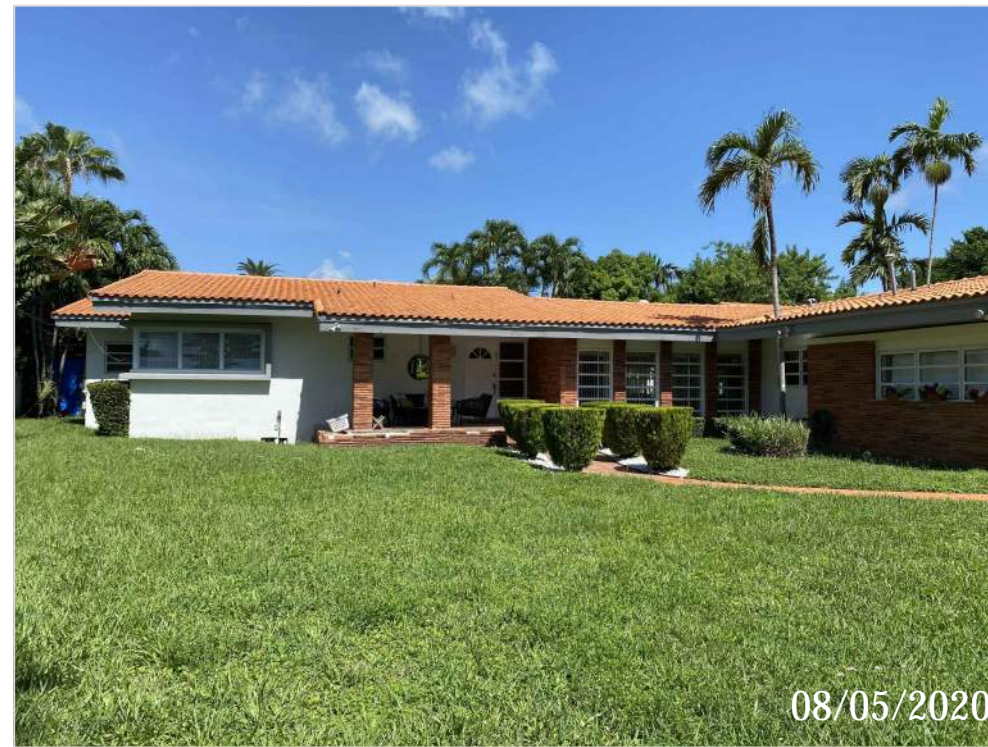
2. 4330 N MICHIGAN AVE FACADE PROPERTY TO THE SOUTH OF PROJECT SUBJECT
