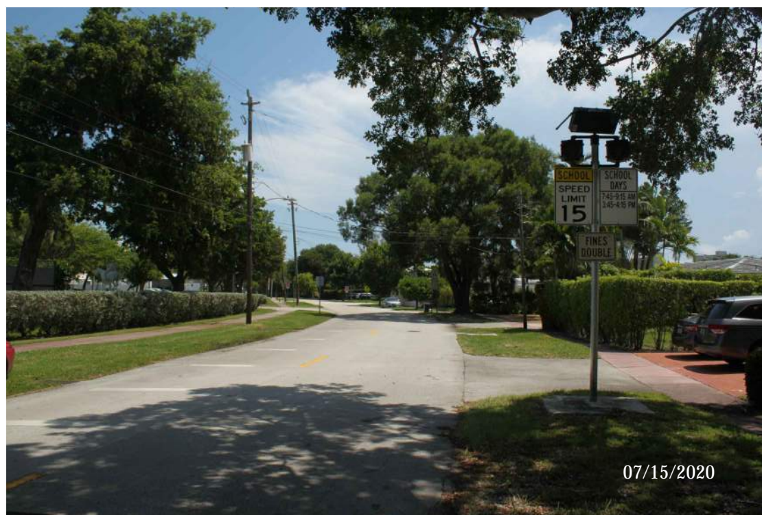
4. SOUTH VIEW FROM FRONT
