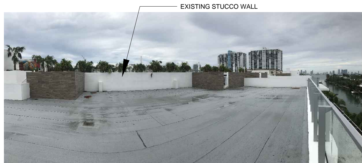
2. ROOF LOOKING WEST
