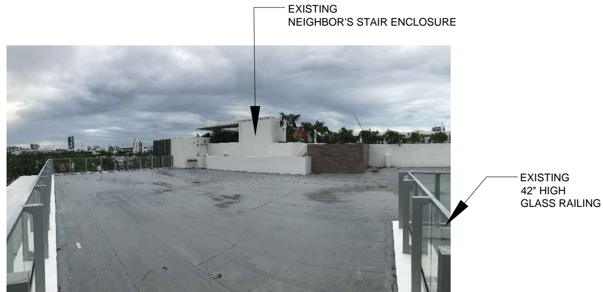
1. ROOF LOOKING EAST
