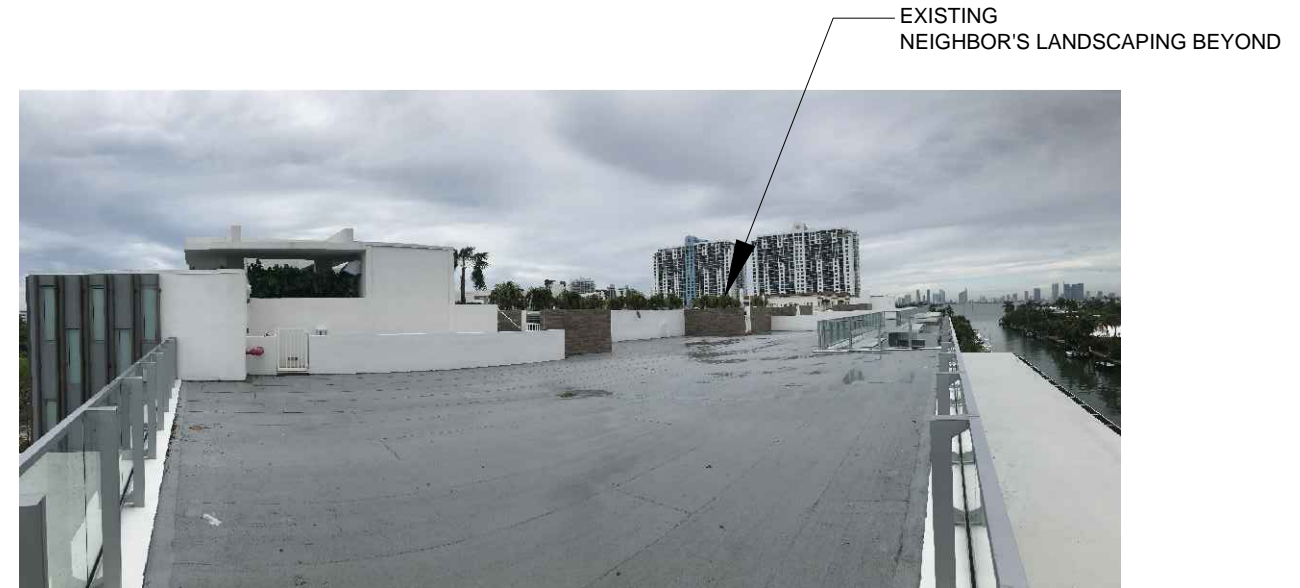
3. ROOF LOOKING NORTH-EAST
