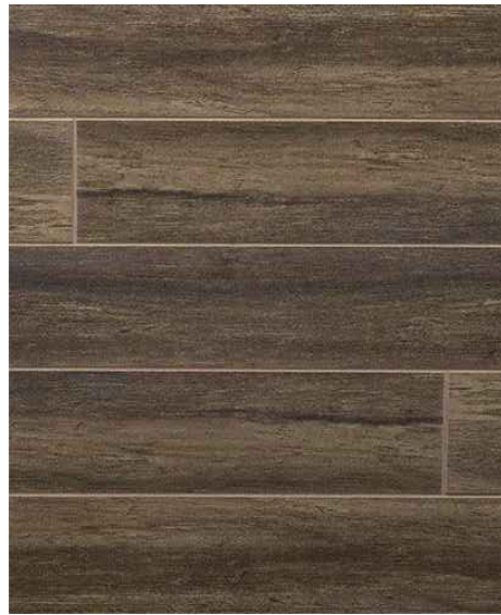
EXISTING PORCELAIN TILE WALLS
