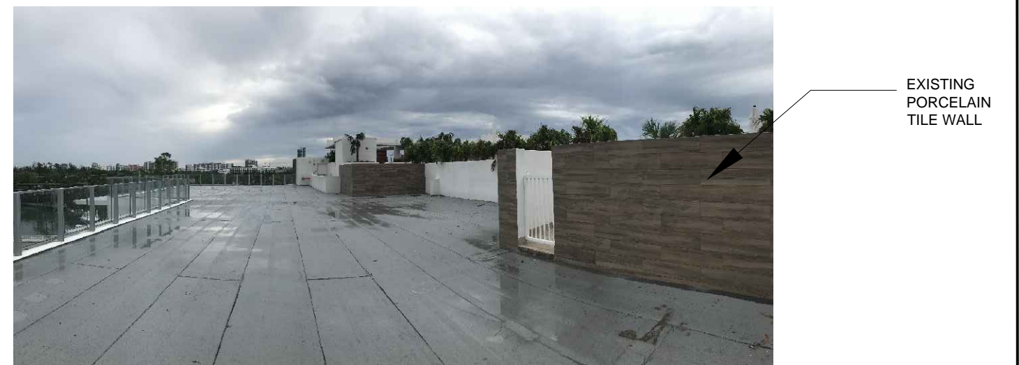
4. ROOF LOOKING NORTH-EAST
