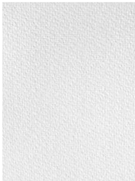
EXISTING STUCCO WALLS
