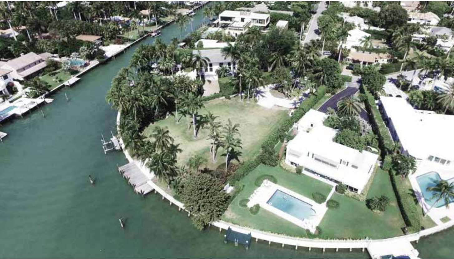
DRONE VIEW LOOKING NORTH EAST
