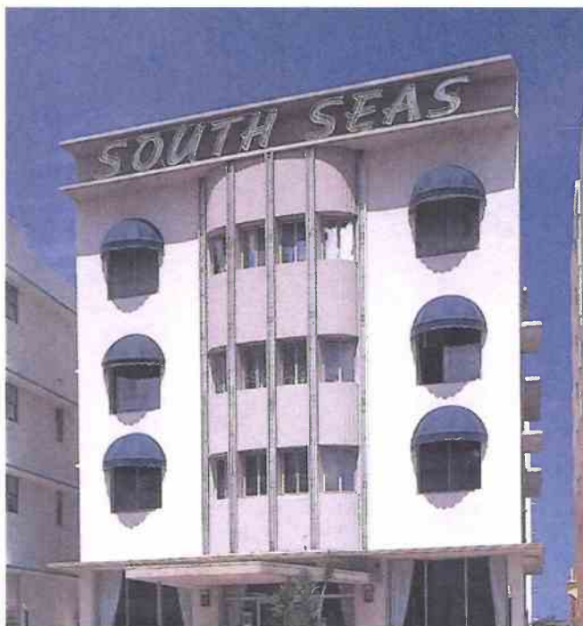
South Seas Hotel, 1988 Photograph 1954 Grossman façade design
