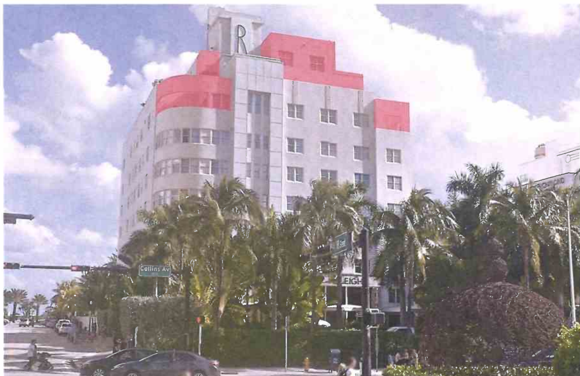
Raleigh Hotel, 2016 Photograph (rooftop additions highlighted in red proposed to be removed)
