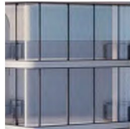
ALUMINUM FRAMES AND GLAZING
