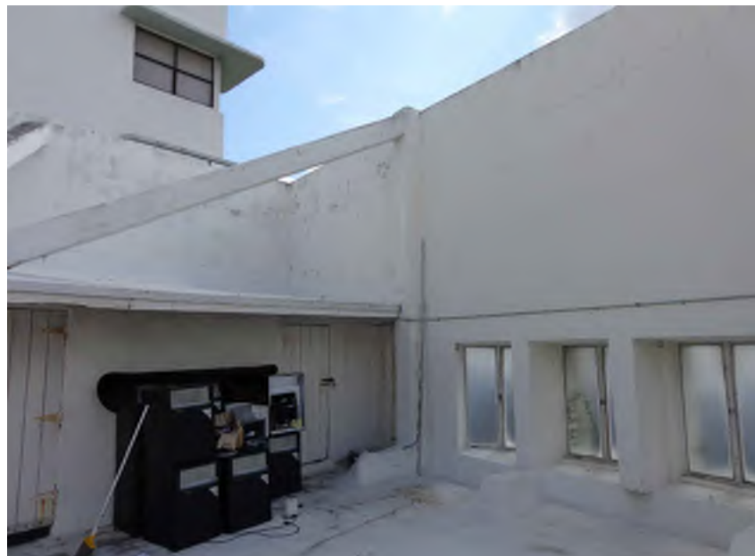
3 SOUTH SEAS- LEVEL FOUR ROOF STORAGE
