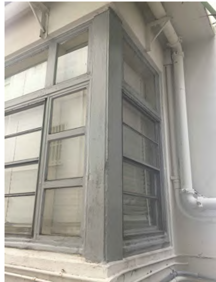
5 THE RICHMOND - SOUTH FACADE ORIGINAL WOOD WINDOW
