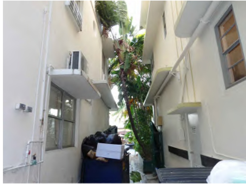
2 WALKWAY BETWEEN RICHMOND & SOUTH SEAS VIEW TOWARD WEST
