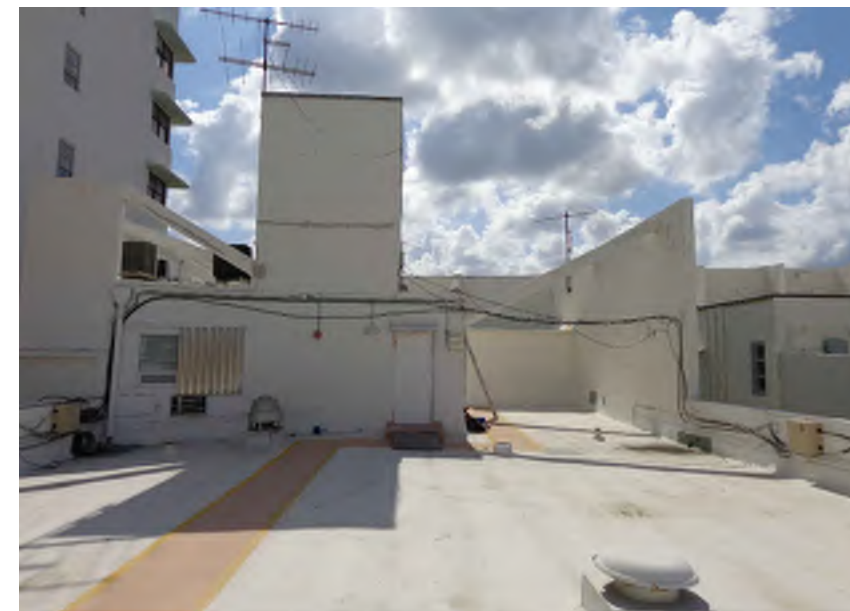
8 SOUTH SEAS - ELEVATOR BULKHEAD
