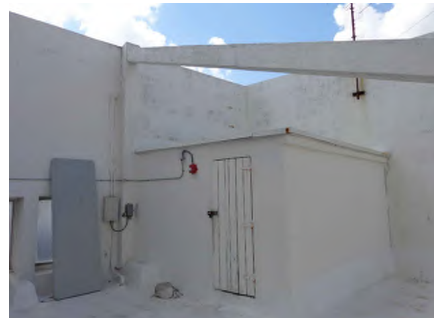
5 SOUTH SEAS- LEVEL FOUR ROOF STORAGE
