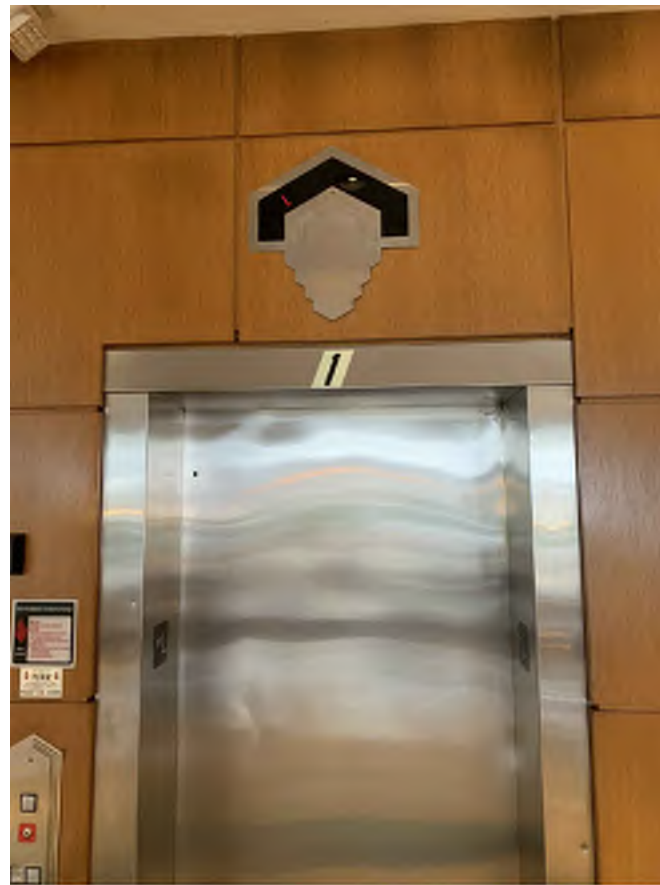
3 THE RICHMOND - ELEVATOR FLOOR INDICATOR DETAIL
