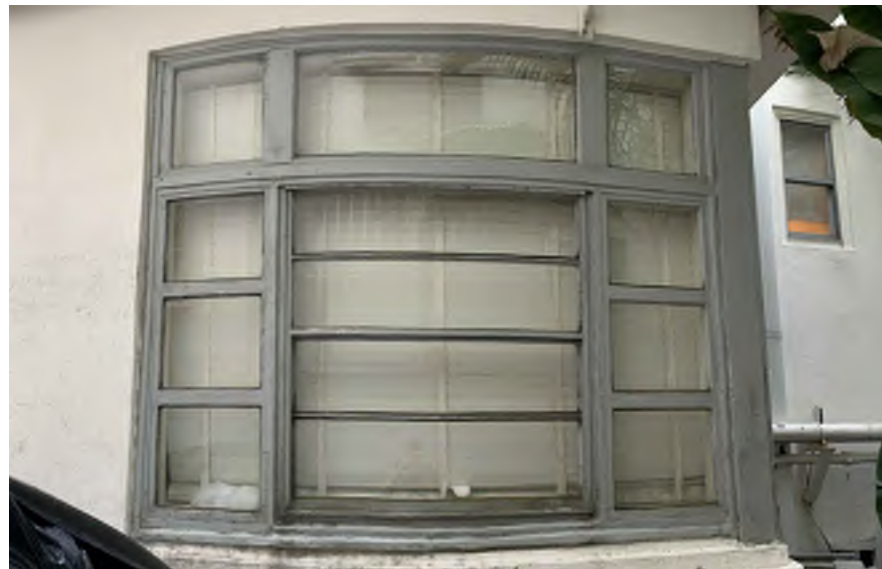
2 THE RICHMOND - SOUTH FACADE ORIGINAL WOOD WINDOW
