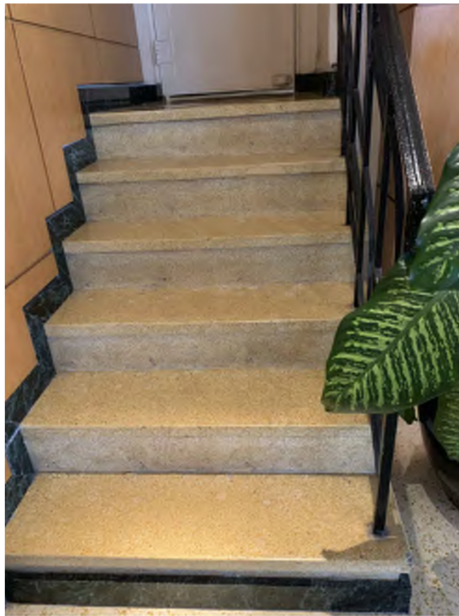
3 THE RICHMOND - LOBBY ORIGINAL TERRAZZO STAIRS
