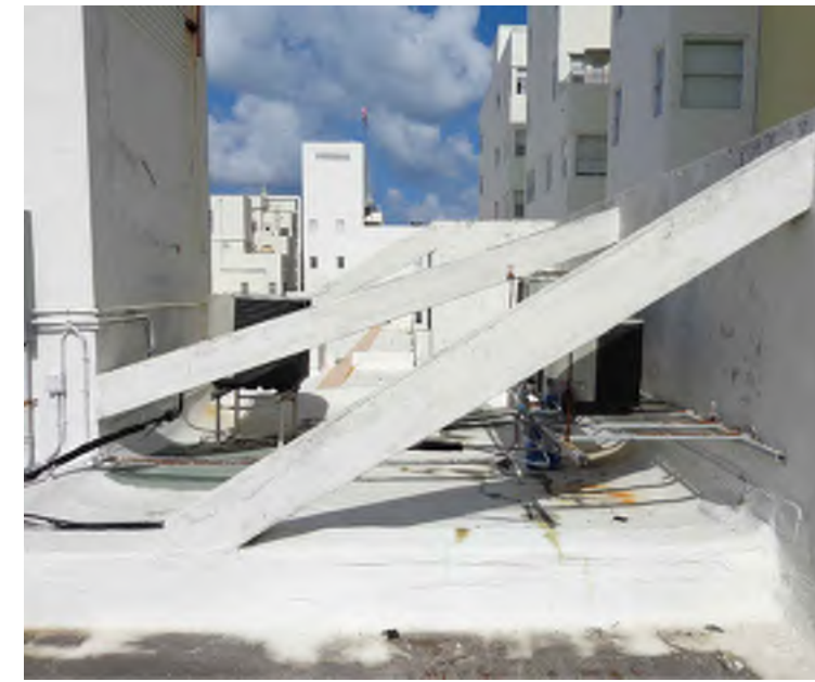
2 SOUTH SEAS- LEVEL FOUR ROOF
