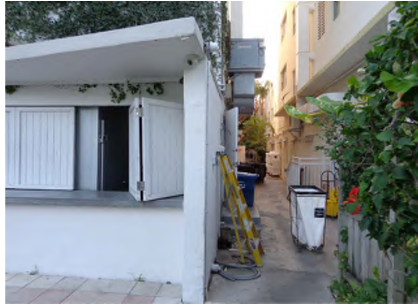
3 WALKWAY BETWEEN RICHMOND & SOUTH SEAS VIEW TOWARD WEST
