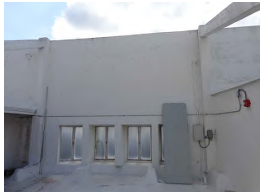
4 SOUTH SEAS- LEVEL FOUR ROOF
