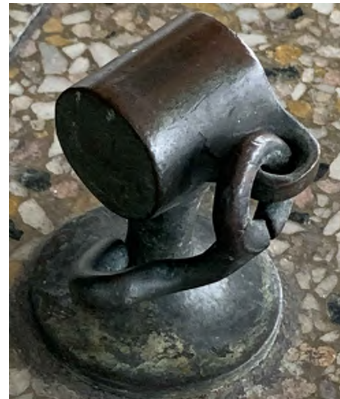
7 THE RICHMOND - FRONT TERRACE DETAIL
