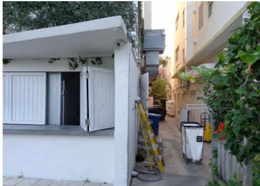
7 THE RICHMOND & SOUTH SEAS BREEZEWAY VIEW FROM EAST
