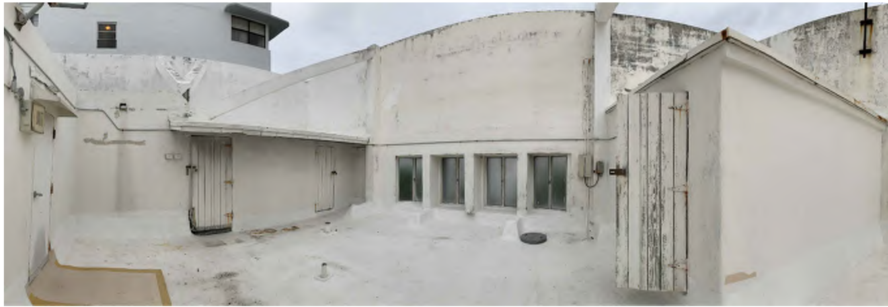
1 SOUTH SEAS- LEVEL FOUR ROOF
