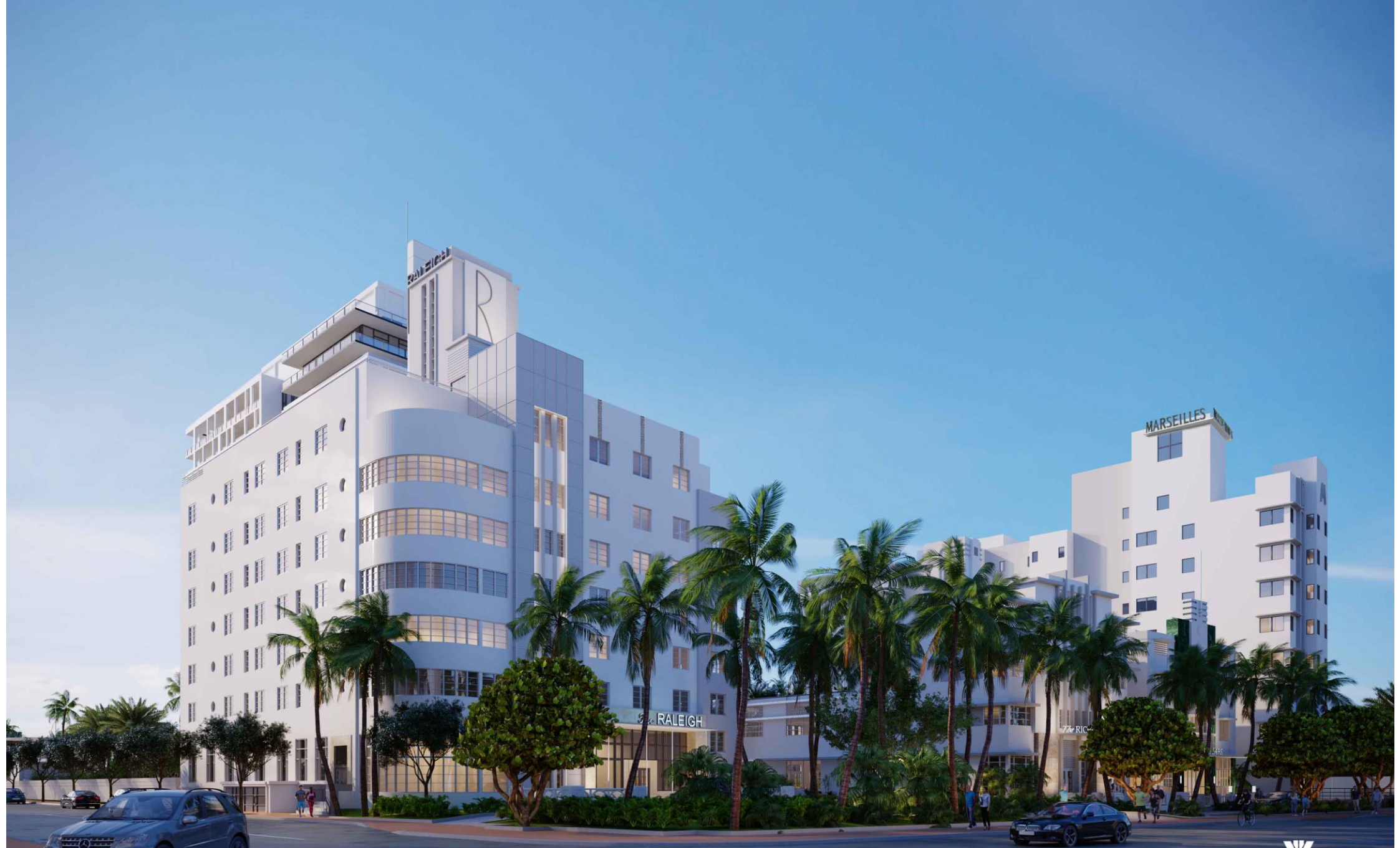
CORNER OF 18 ST AND COLLINS AVE LOOKING TO THE SOUTH-EAST AT RESTORED RALEIGH FAÇADE
