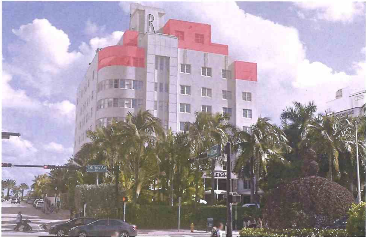
Raleigh Hotel, 2016 Photograph (rooftop additions highlighted in red proposed to be removed)
