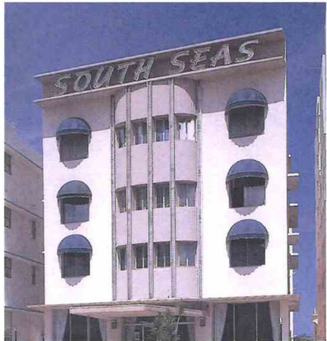
South Seas Hotel, 1988 Photograph 1954 Grossman façade design
