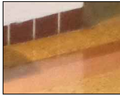
3 EXISTING WOOD PANELING
