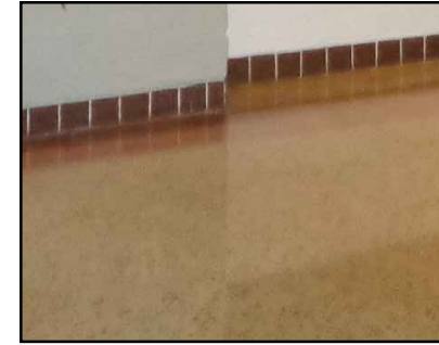
3 HISTORIC TERRAZZO FLOORING AND BASEBOARD
