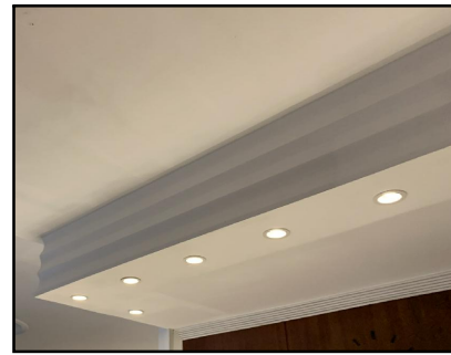
3 HISTORIC RECEPTION DROP-CEILING FEATURE
