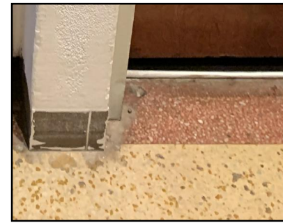
4 HISTORIC TERRAZO FLOORING AND BASEBOARD
