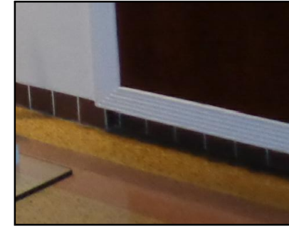
4 HISTORIC TERRAZO FLOORING AND BASEBOARD
