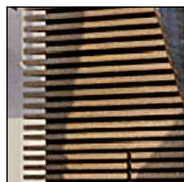
ALUMINUM SCREEN CLADDING
