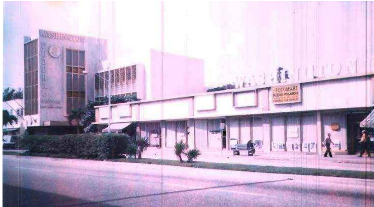
1970 WASHINGTON AVENUE FACADE SHOWING ORIGINAL CONFIGURATION AND MATERIALS
