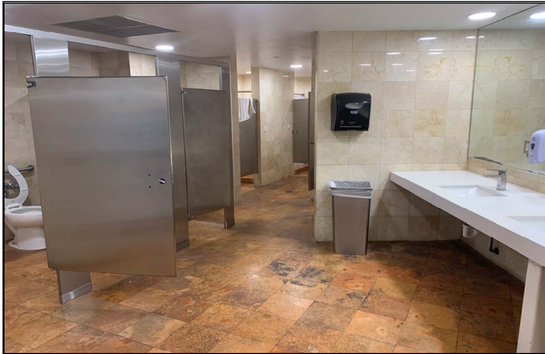
INTERIOR VIEW OF MEN'S BATHROOM AND SHOWERS
