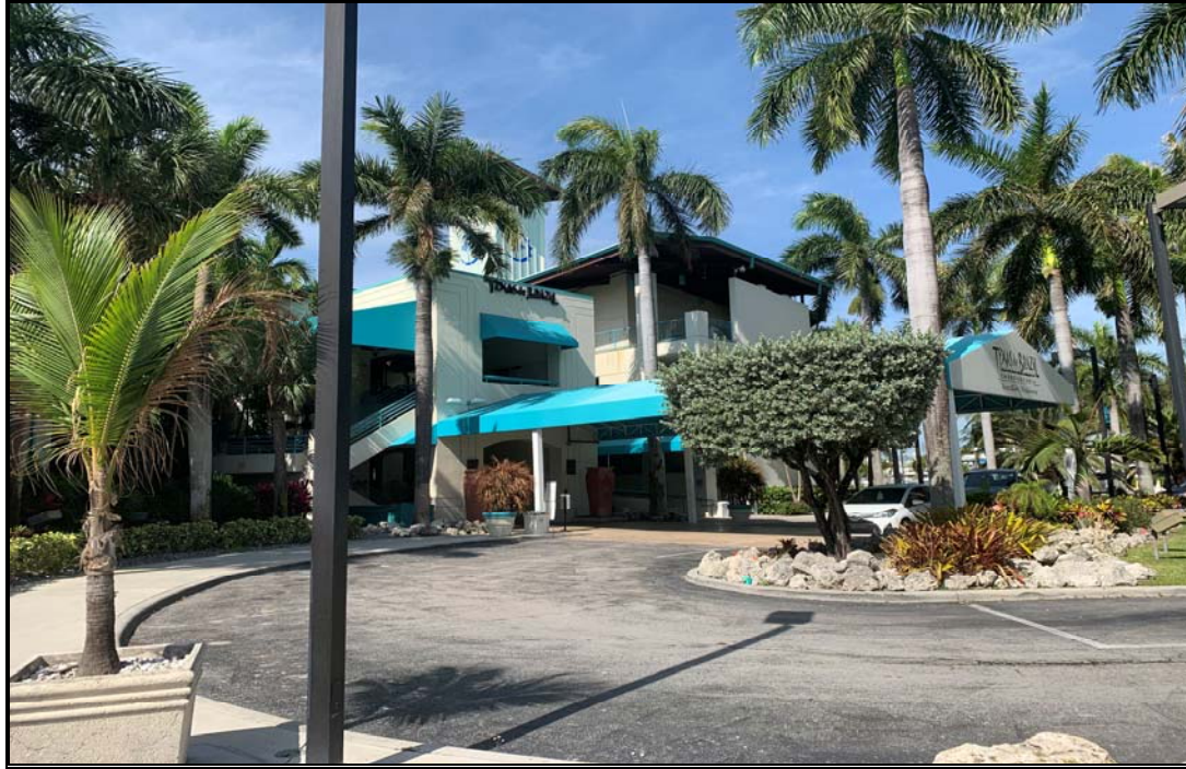
VIEW LOOKING SOUTHWEST AT THE CORE BUILDING
