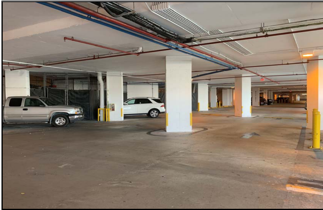
NORTH PARKING GARAGE
