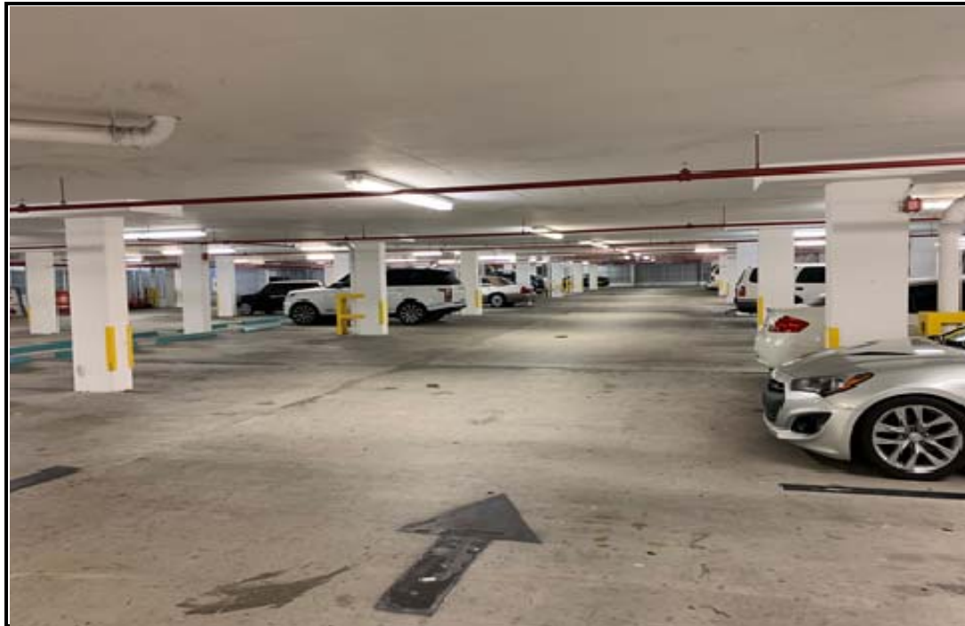
SOUTH PARKING GARAGE
