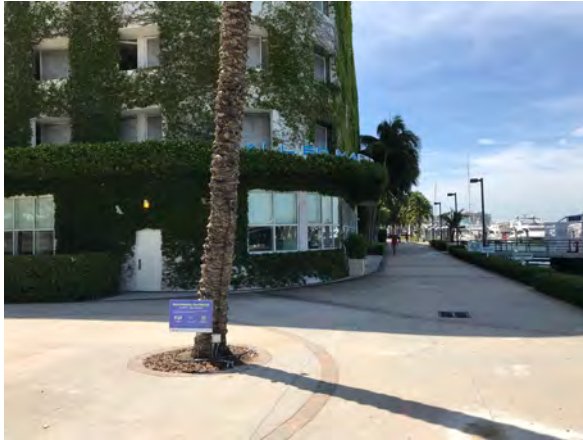
Photo 13 – Allied Marine Office - Exterior
