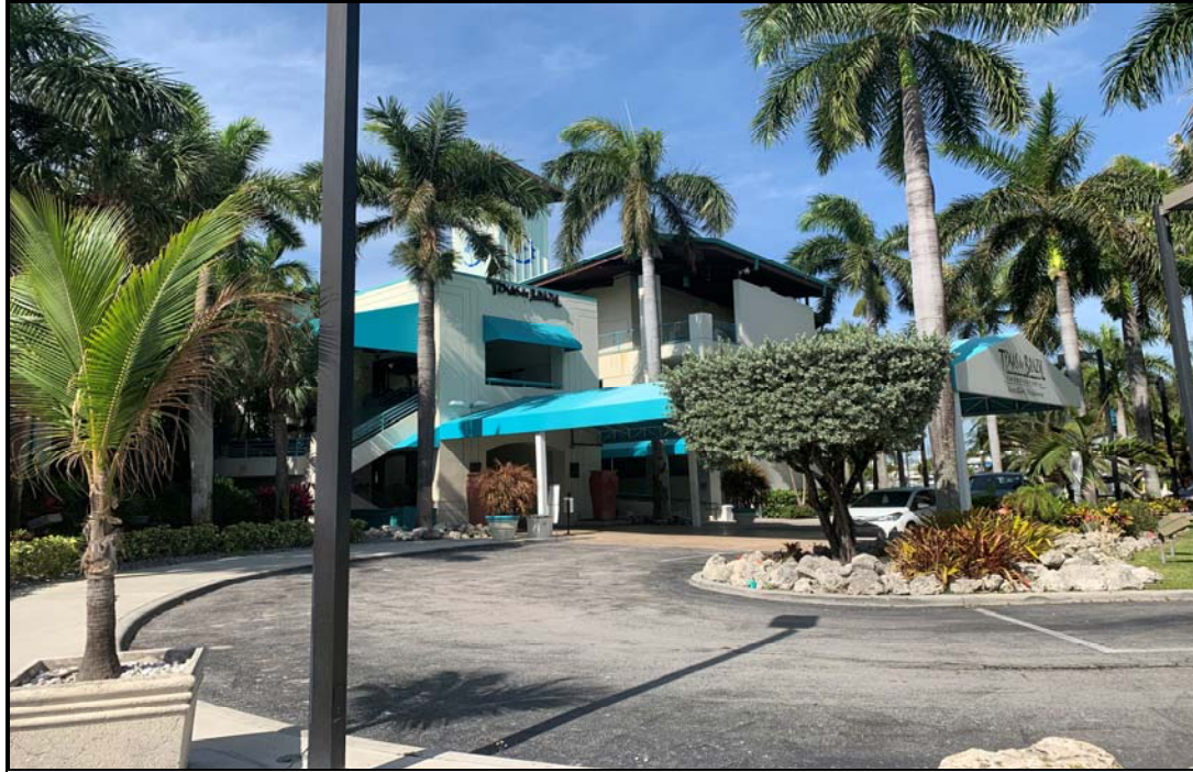
VIEW LOOKING SOUTHWEST AT THE CORE BUILDING
