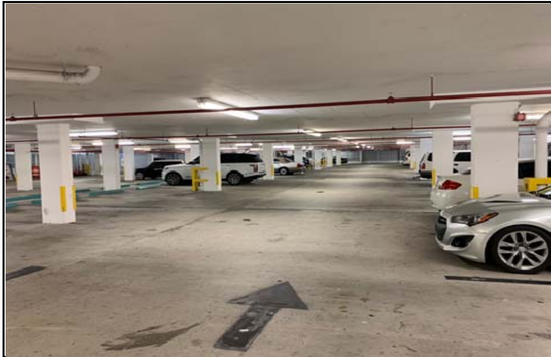
SOUTH PARKING GARAGE
