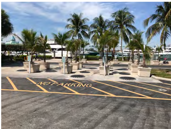
Photo 17 – Fuel Tank Farm (USTs)
