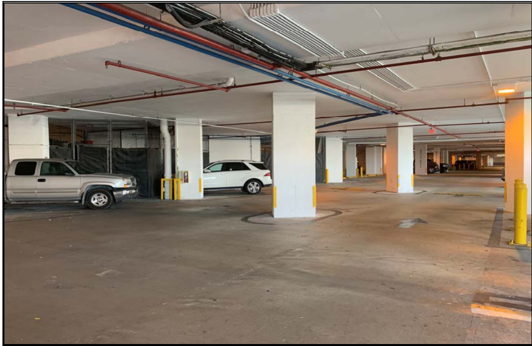
NORTH PARKING GARAGE
