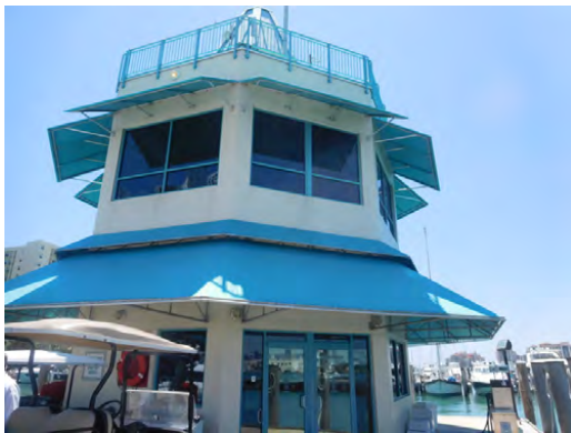
PHOTO #5 FUEL PAYMENT/OFFICE BUILDING
