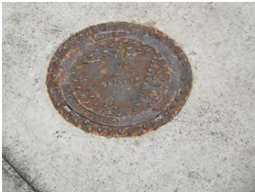
PHOTO #39 ABANDONED MONITORING WELL
