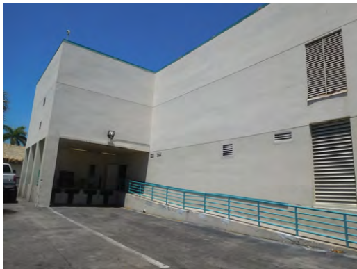
PHOTO #3 SOUTH ELEVATION, MAIN BUILDING
