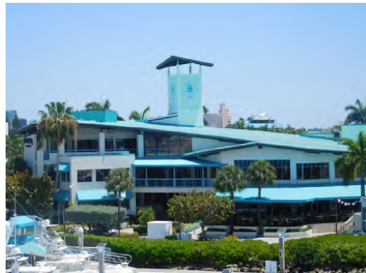
PHOTO #4 WEST ELEVATION, MAIN BUILDING
