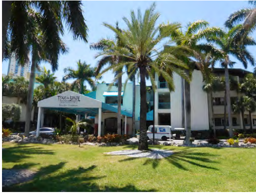
PHOTO #1 NORTH ELEVATION, MAIN BUILDING
