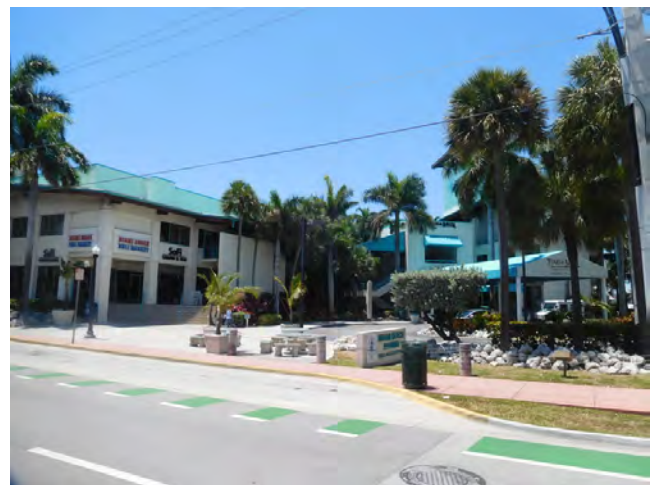
East elevation, main building
