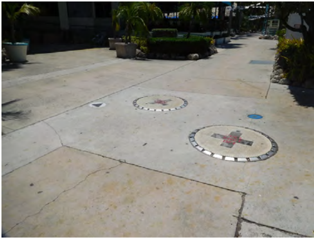
Fuel line sumps
