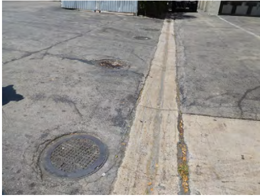
PHOTO #37 GREASE TRAPS
