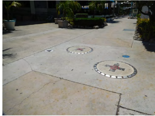
PHOTO #26 FUEL LINE SUMPS
