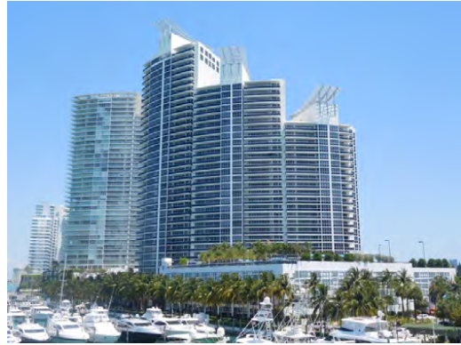
PHOTO #44 ADJACENT NORTH - CONDOMINIUMS
