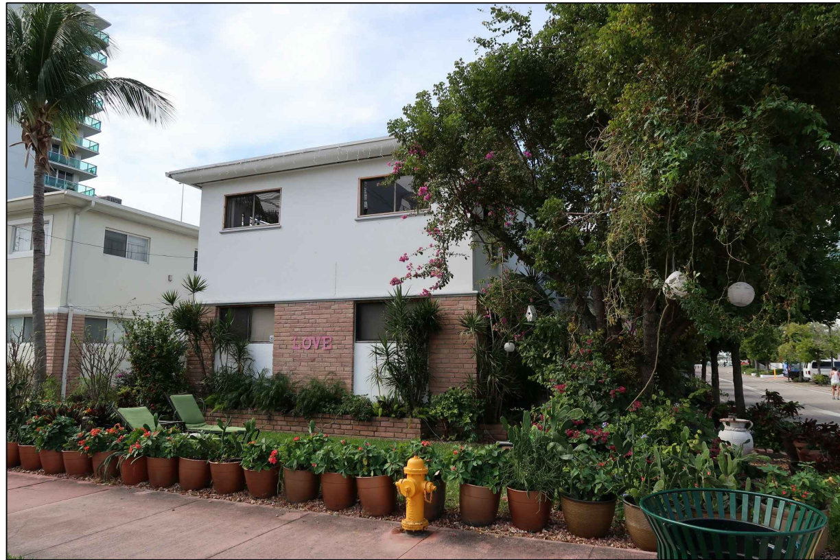
PROPERTY 8 (WEST AVE VIEW) N.T.S.
