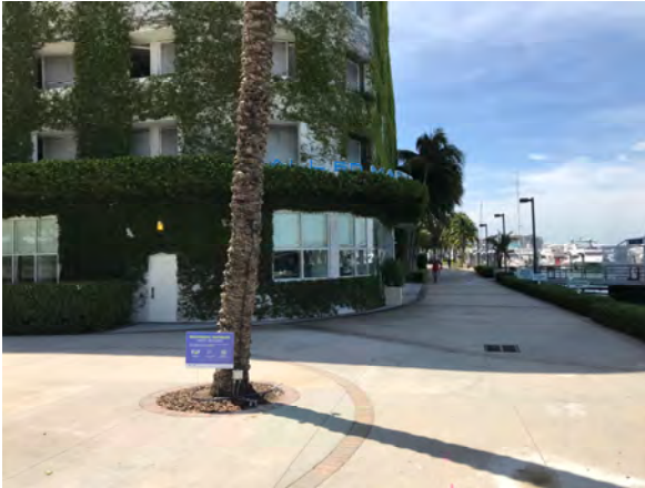
Photo 13 – Allied Marine Office - Exterior
