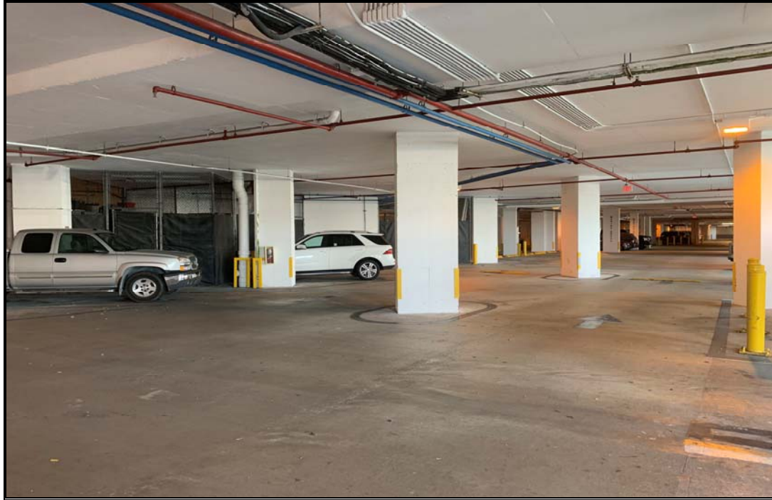
NORTH PARKING GARAGE
