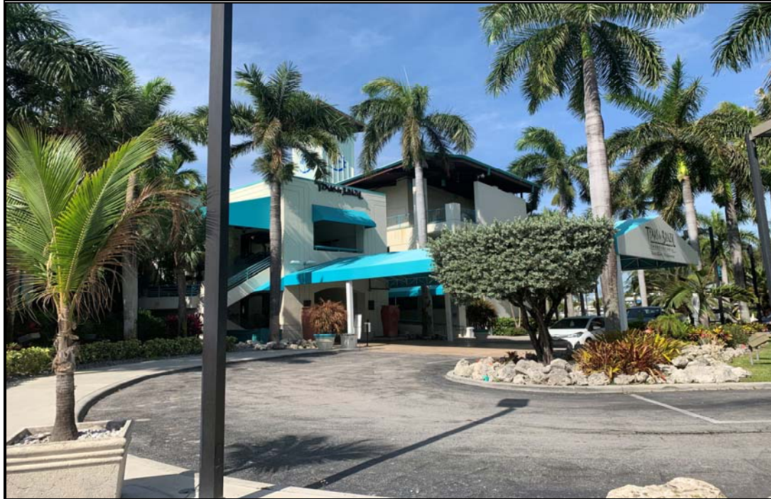
VIEW LOOKING SOUTHWEST AT THE CORE BUILDING
