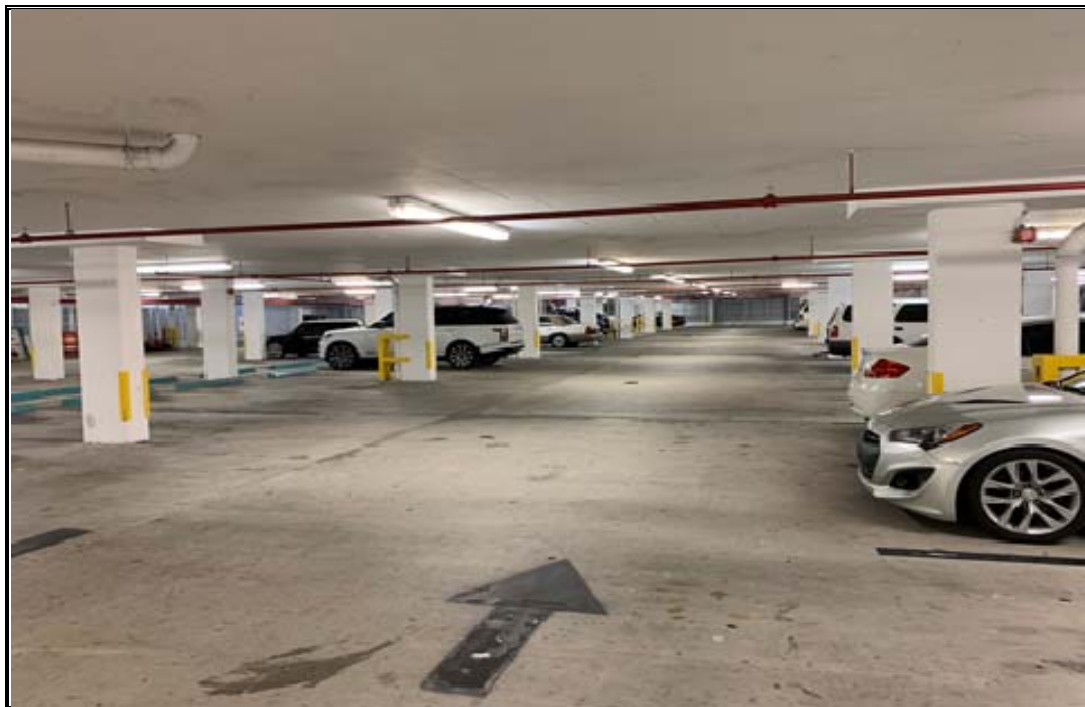
SOUTH PARKING GARAGE
