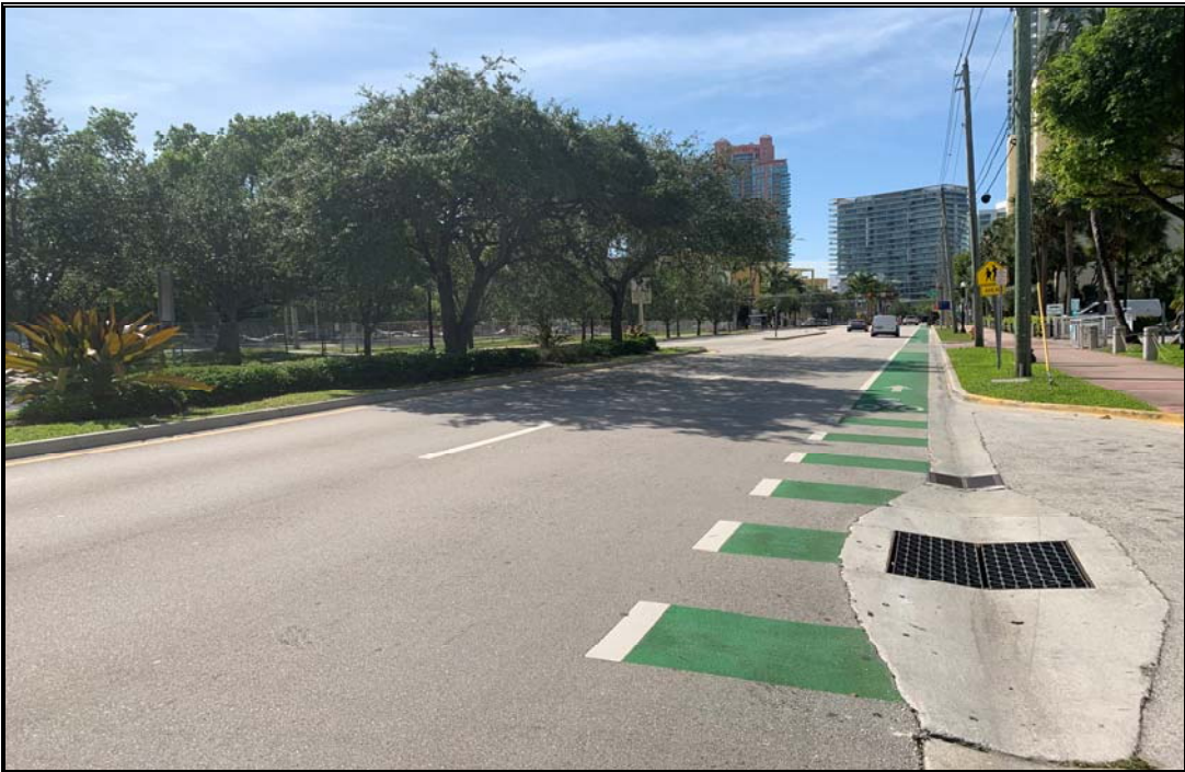
STREET SCENE – VIEW SOUTH ALONG ALTON ROAD
