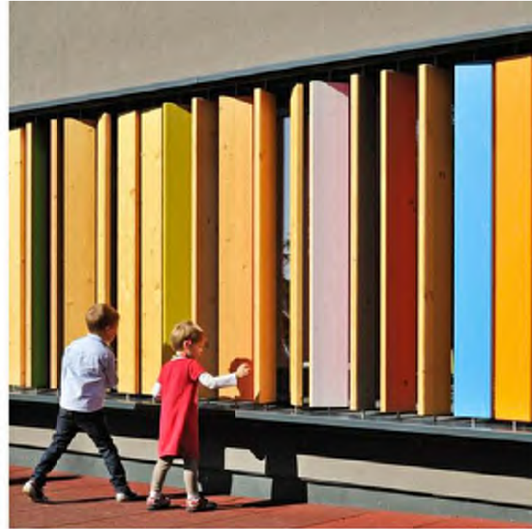
COLORED LOUVERS at the drop off as well as the ground floor of new addition
