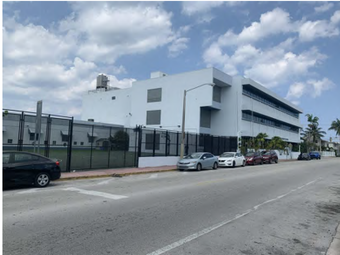
(1) VIEW FACING NORTHEAST ON 77th STREET
