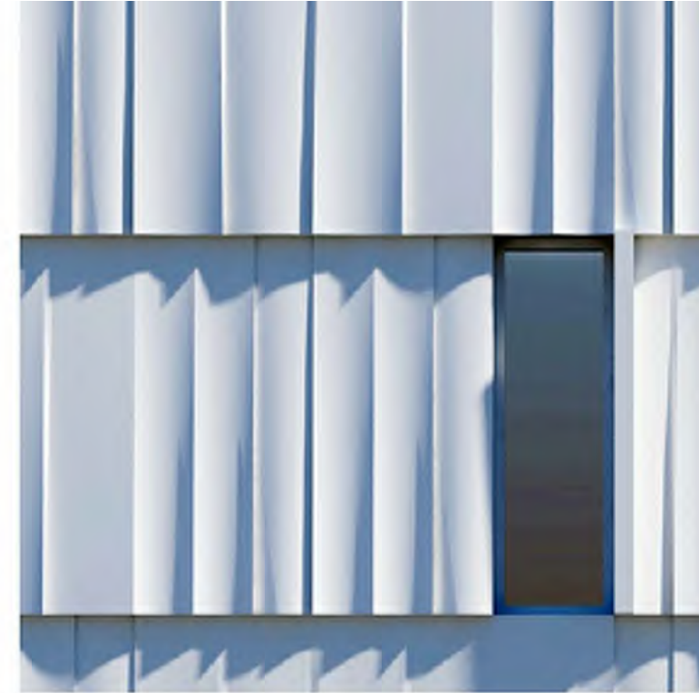
SCULPTURAL PRECAST PANELS at the second and third floors of new addition
