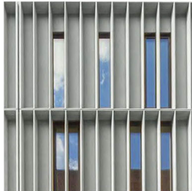
VERTICAL CONCRETE FINES at the lower volume of new addition
