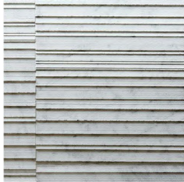
HORIZONTAL STUCCO BANDS at the transition between existing school and new addition
