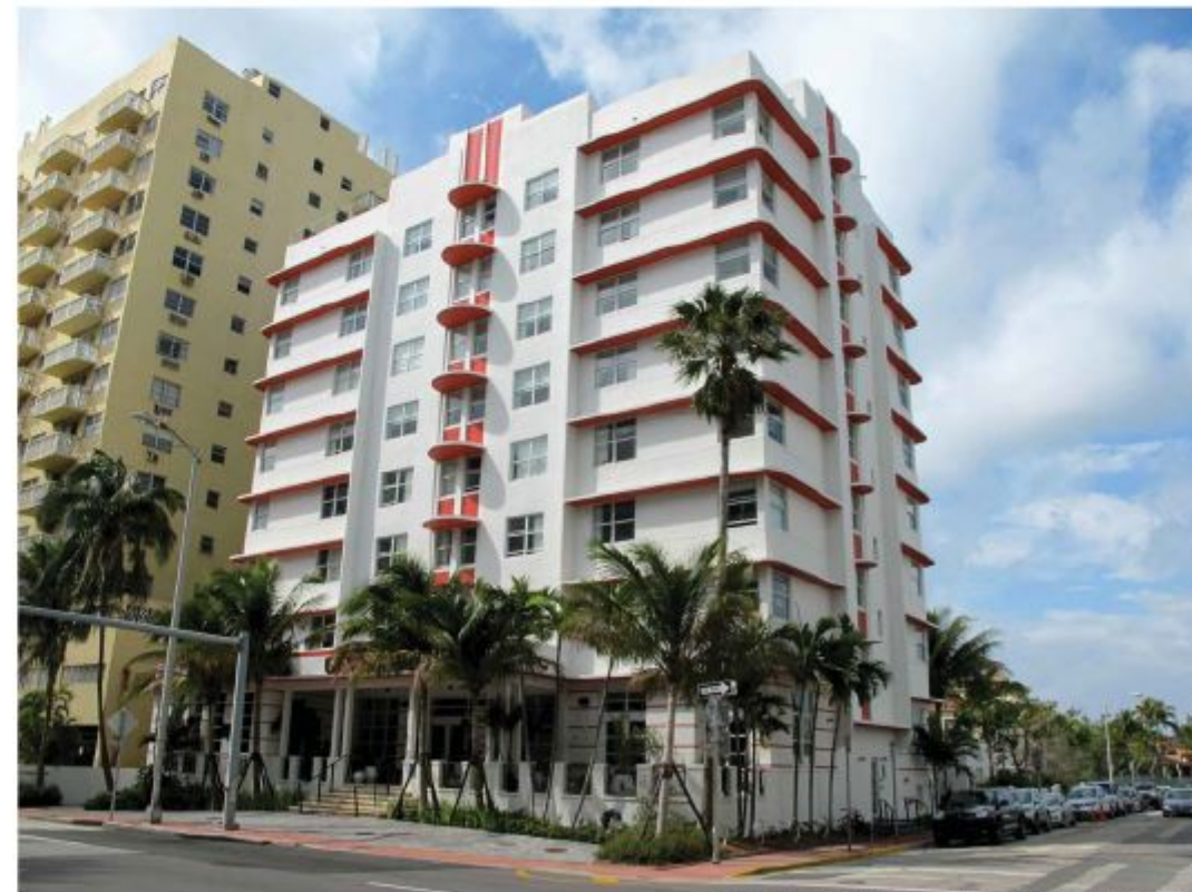
RENDALE HOTEL, POST-IMPROVEMENTS (2019)
