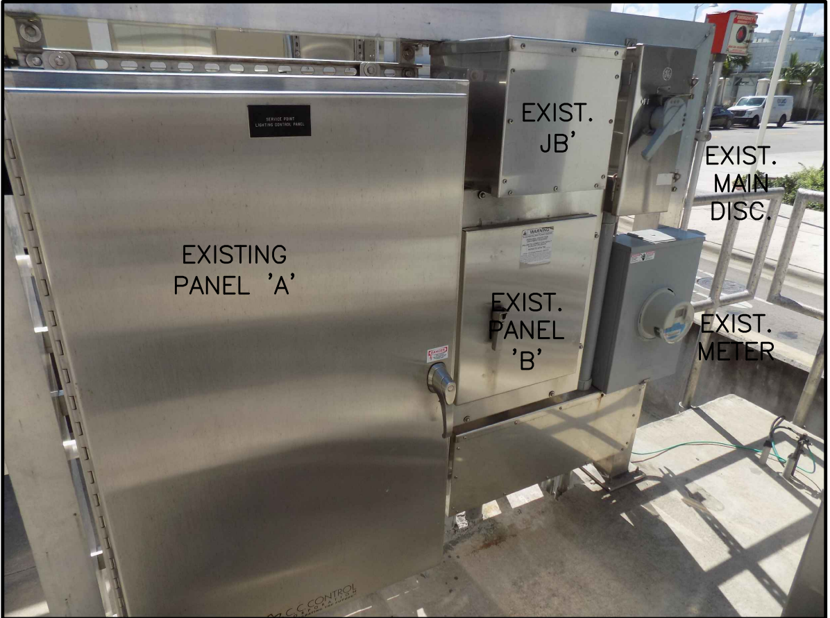
EXISTING PANEL 'A' AND SERVICE POINT
