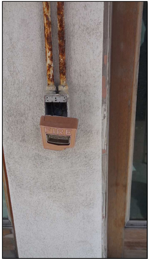
Figure 19: Exposed electrical
