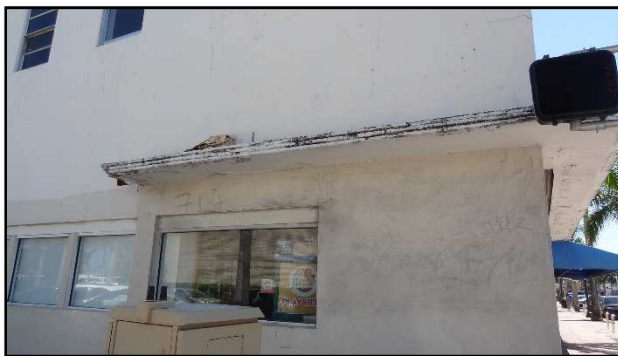
Figure 11: Crumbling eyebrow along Collins Avenue
