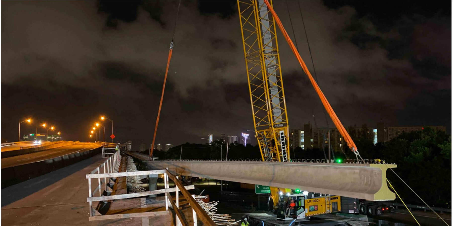
Setting beam on SR 836 over the northbound NW 17 Avenue Ramp
