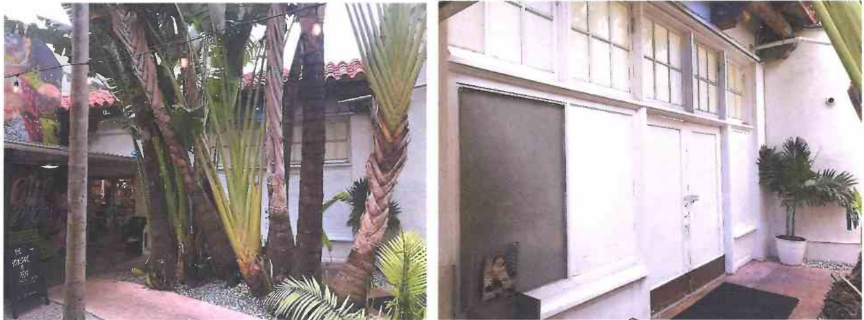
El Patio Building, 2019
