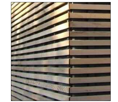
G Wood Trellises
