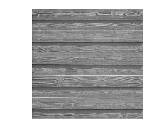
A Exposed Concrete
