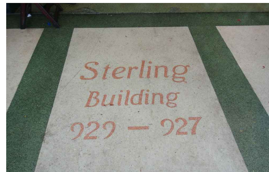
EXISTING GROUND LEVEL FLOORING: IMAGE 1
