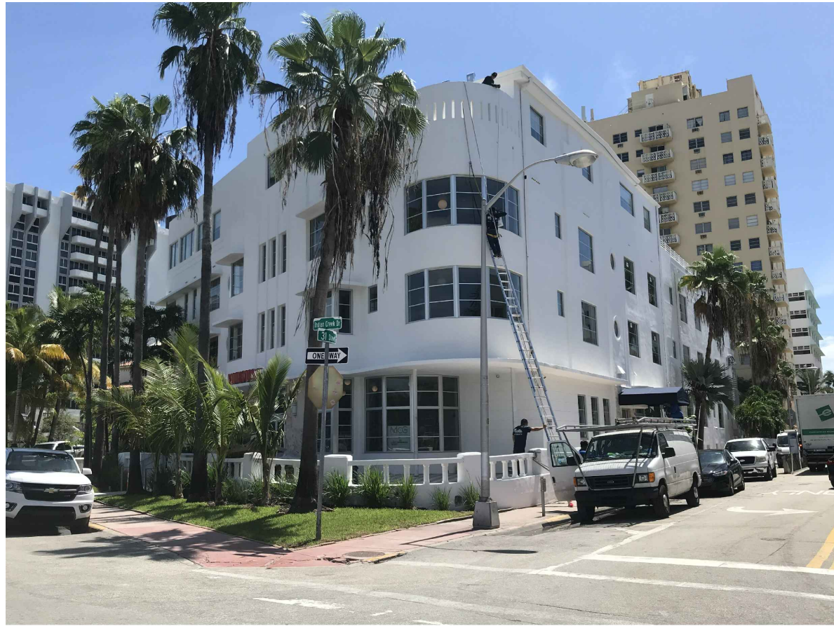
FRONT FACADE ON THE CORNER OF INDIAN CREEK AND 31ST STREET
