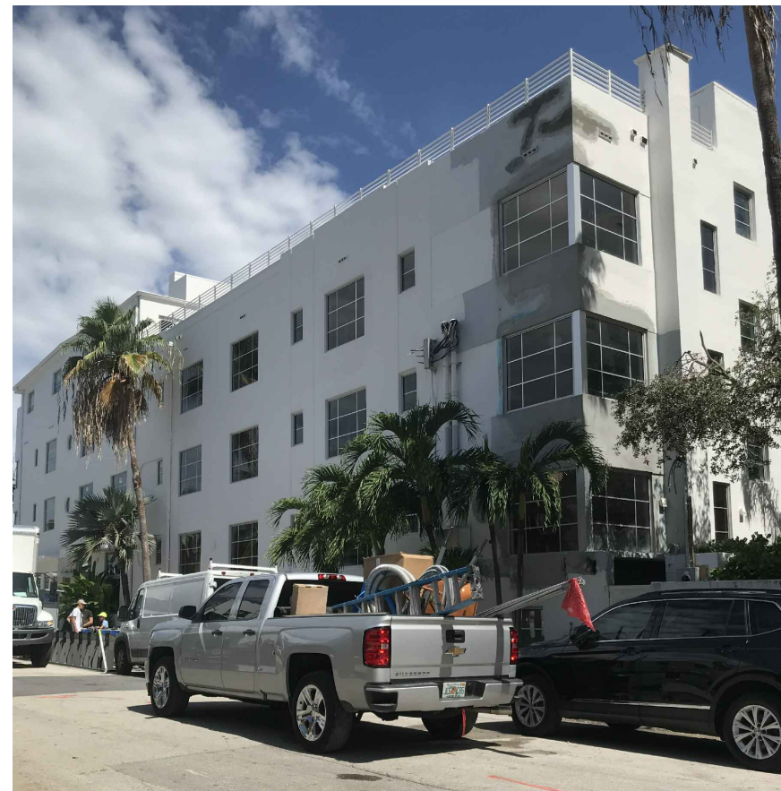
VIEW NEXT TO PARKING LOT
