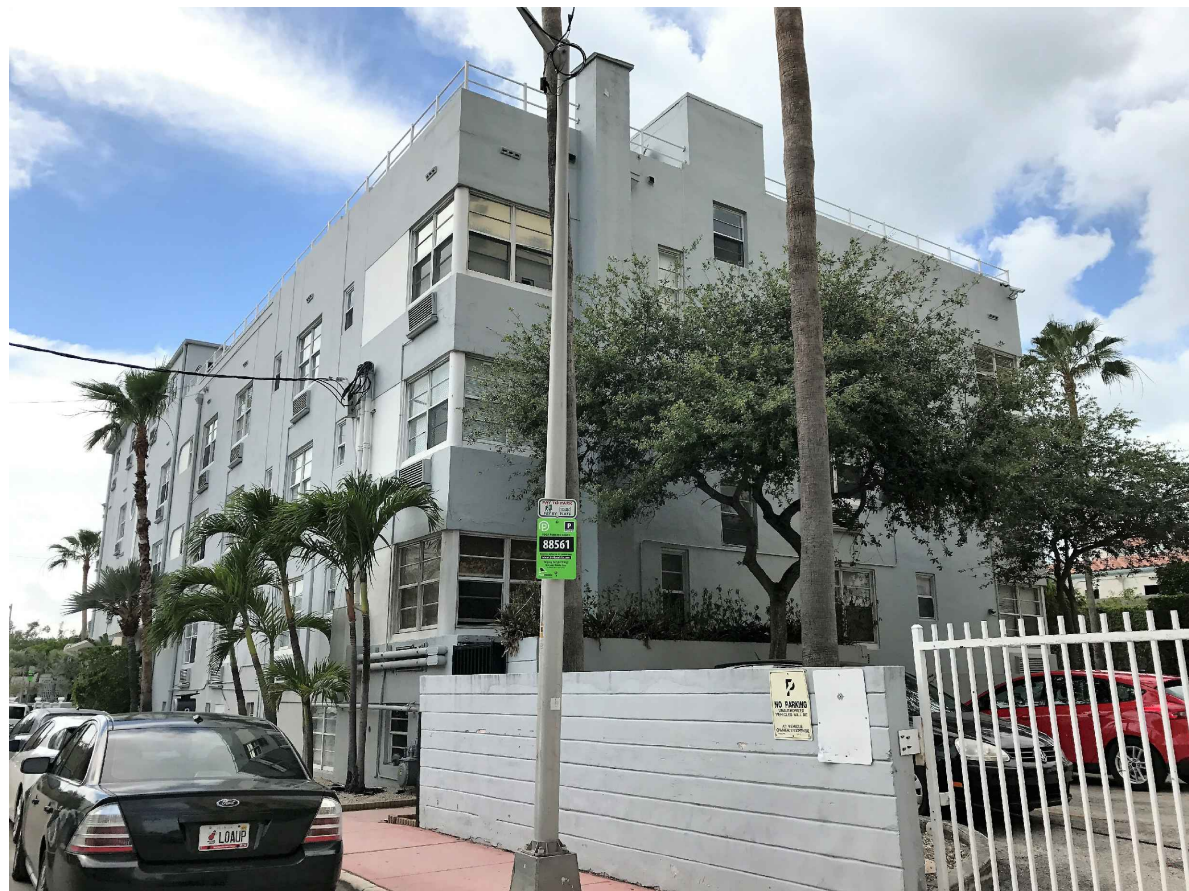
REAR FACADE FACING EAST
