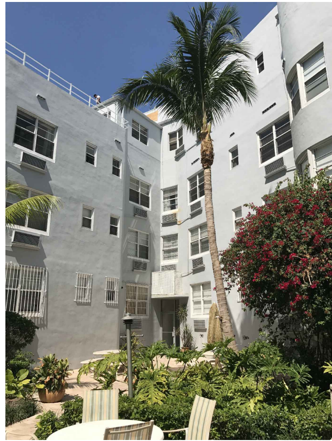
VIEW FACING EAST ON INDIAN CREEK
