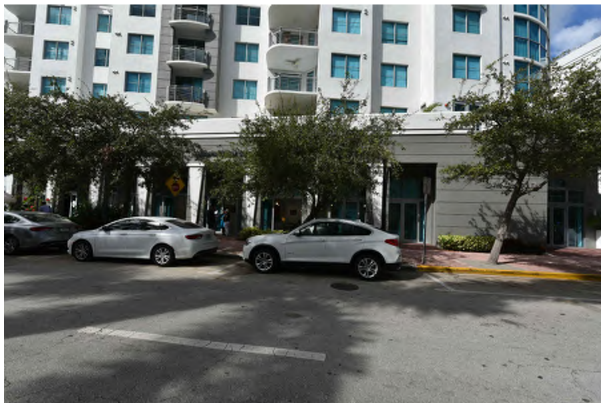
EXISTING VIEW OF SUBJECT AND NORTHERLY NEIGHBORING RETAIL FROM WASHINGTON AVE.
