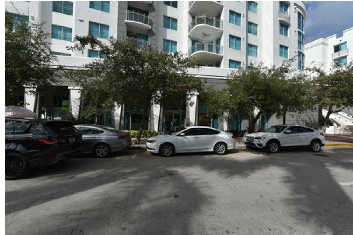
EXISTING VIEW OF SUBJECT AND SOUTHERLY NEIGHBORING RETAIL FROM WASHINGTON AVE.
