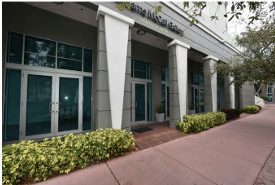
EXISTING VIEW OF WASHINGTON AVE ARCADE LOOKING NORTH
