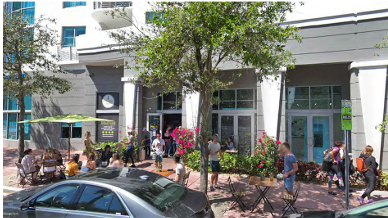
ENLARGED VIEW OF PURA VIDA, NEIGHBORING SPACE TO THE SOUTH. REFER TO SHT P-101 FOR "NEIGHBORING RETAIL" PHOTOGRAPHS.
