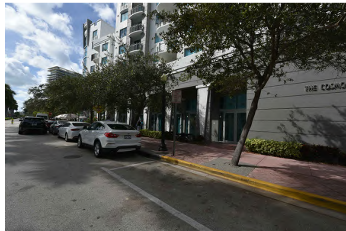
EXISTING VIEW OF MOST-NORTHERLY NEIGHBORING RETAIL FROM WASHINGTON AVE.
