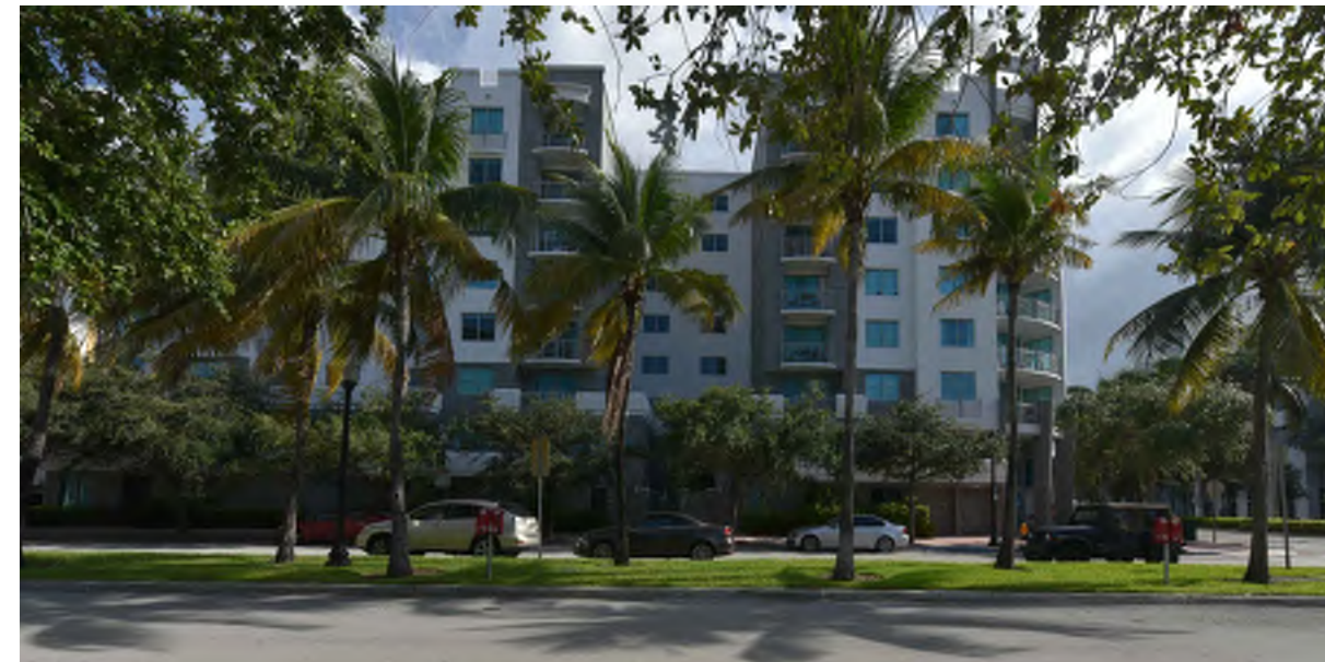
EXISTING VIEW FROM 1ST STREET, SOUTH ELEVATION; LOOKING NORTH.
