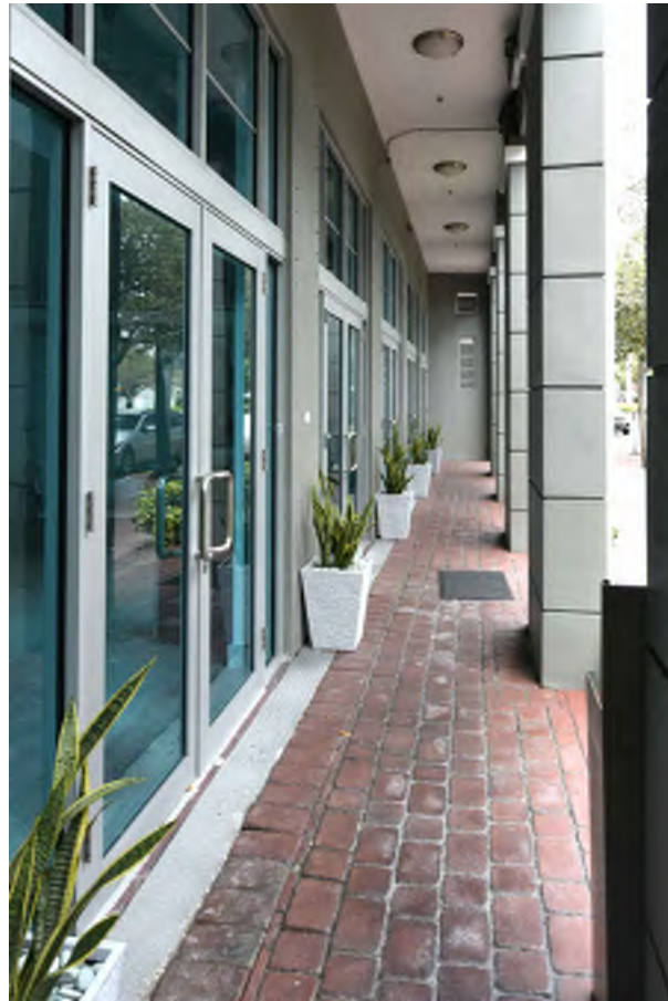
EXISTING VIEW OF WASHINGTON AVE ARCADE LOOKING NORTH
