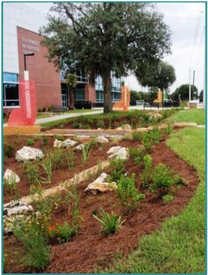
Bioretention facility at the University of Florida Southwest Recreation Center
