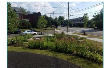
Bioretention facility in unused triangular open space that was converted to a public park
