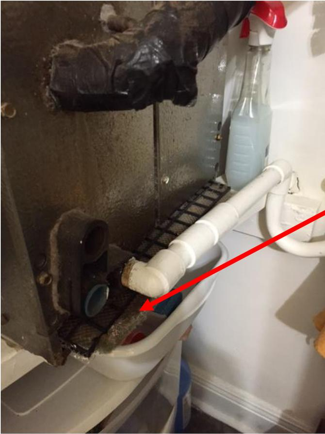
A/C air filter in very poor condition; tenant claims no replacement provided
