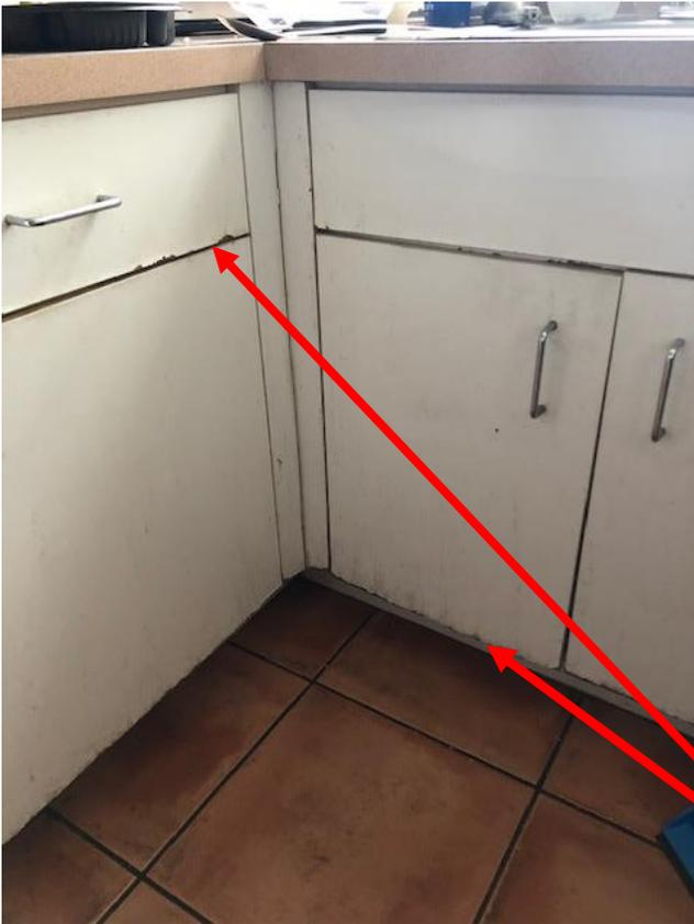
The kitchen cabinets are in poor condition fraying at the end with peeling paint.
