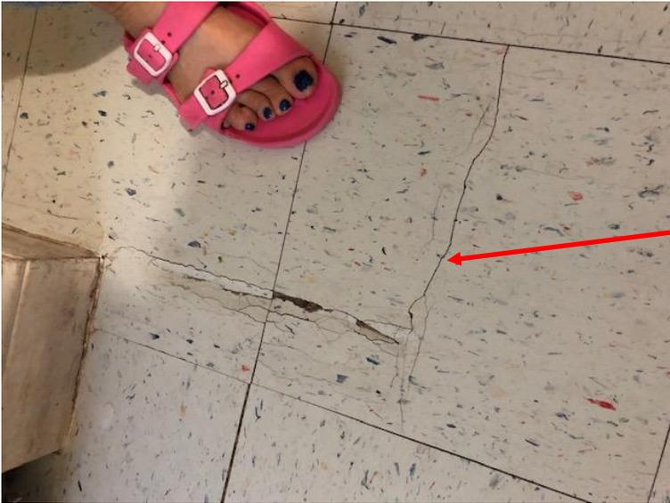
Floor is buckling within unit causing tiles to break
