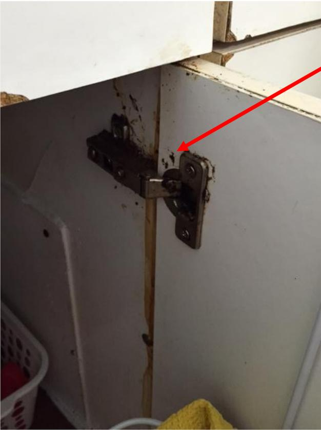
Kitchen cabinets improperly hung and in poor condition
