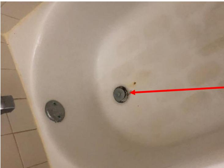
Rusted tub fixture that does not seal properly
