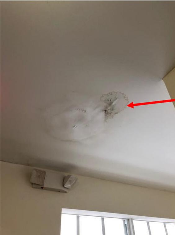
Water stains, peeling paint, and what appears mold in common area in upper floor
