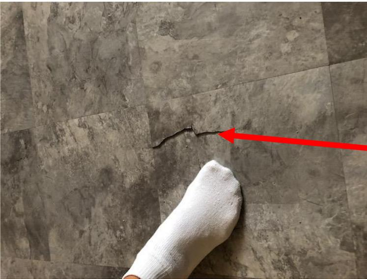
Floor at center of living room is buckling and has resulted in broken tile.
