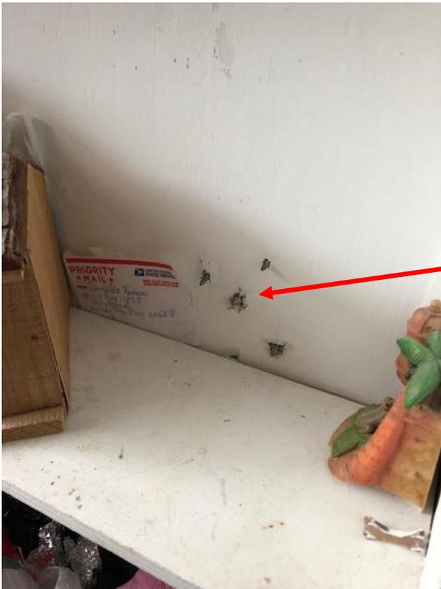
There are screws from the bathroom wall into the kitchen fully exposed and creating a hazard.
