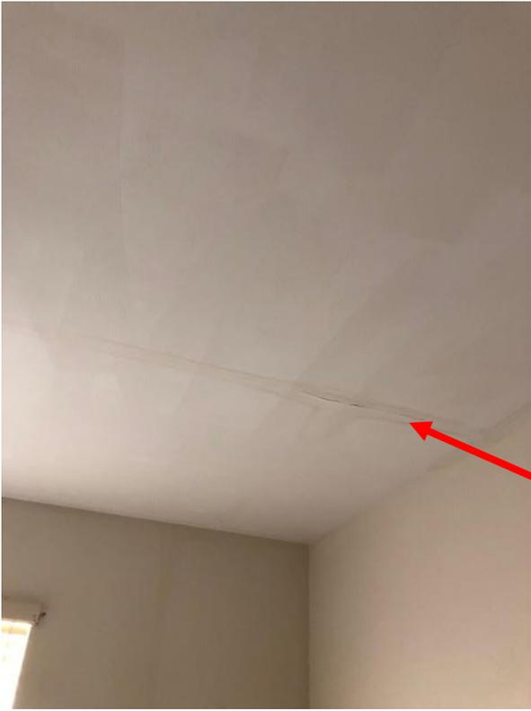
Water damage; stains; dry wall seams exposed
