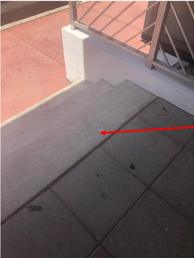
Rivets pose trip hazard at top step next to wheelchair lift
