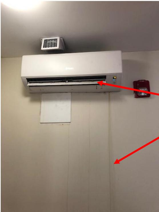
Common area AC unit is dirty and is leaking down walls creating stains
