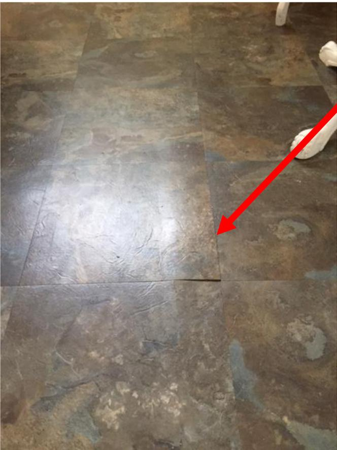
Tiles in bedroom are lifting or cracked from buckling
