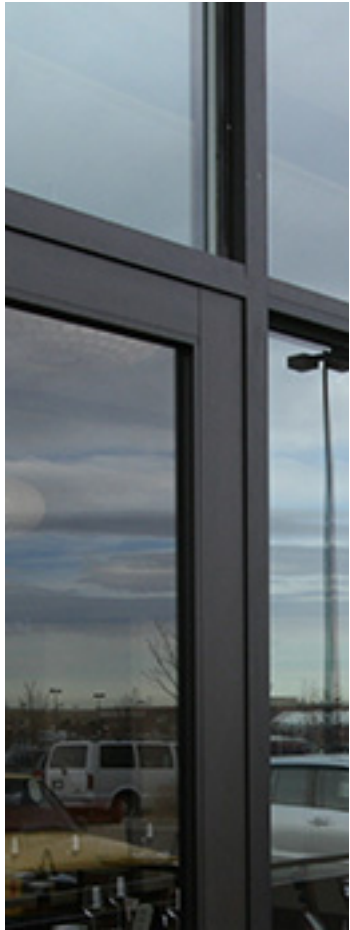
black aluminum framed impact glazing and doors
