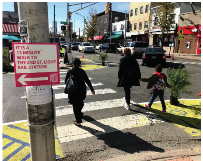
Curb extensions at the busy intersection of Sip and Bergen shortened crossing distances, added color pop, and made pedestrians more visible to turning motorists.
