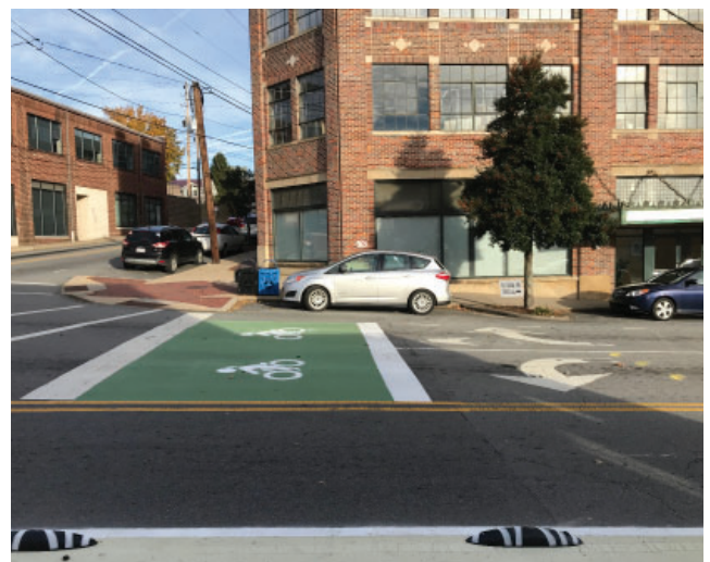
The .3-mile corridor was lined with various planters and bollards to protect pedestrians and cyclists in the new shared path (top).
