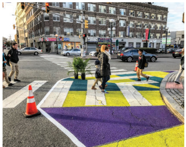
Curb extensions at Westside and Belmont reduced crossing distances by 40%.
