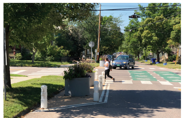
Design Standards in the Guide contain specs and application examples for a wide range of street design elements, like curb extensions (above), which have already been implemented by Burlington Public Works along priority corridors identified in the plan btv walk/bike master plan.
