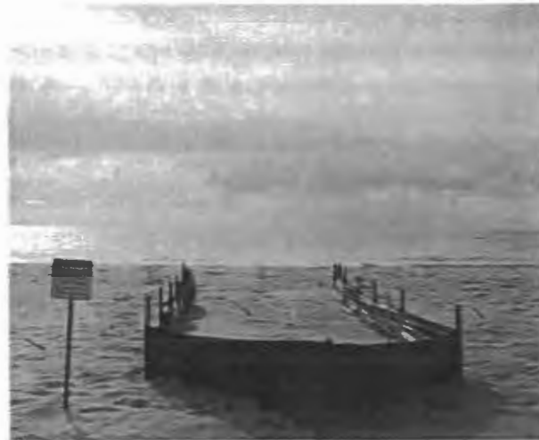
SILT FENCING - CAPE HATTERAS NATIONAL SEASHORE
