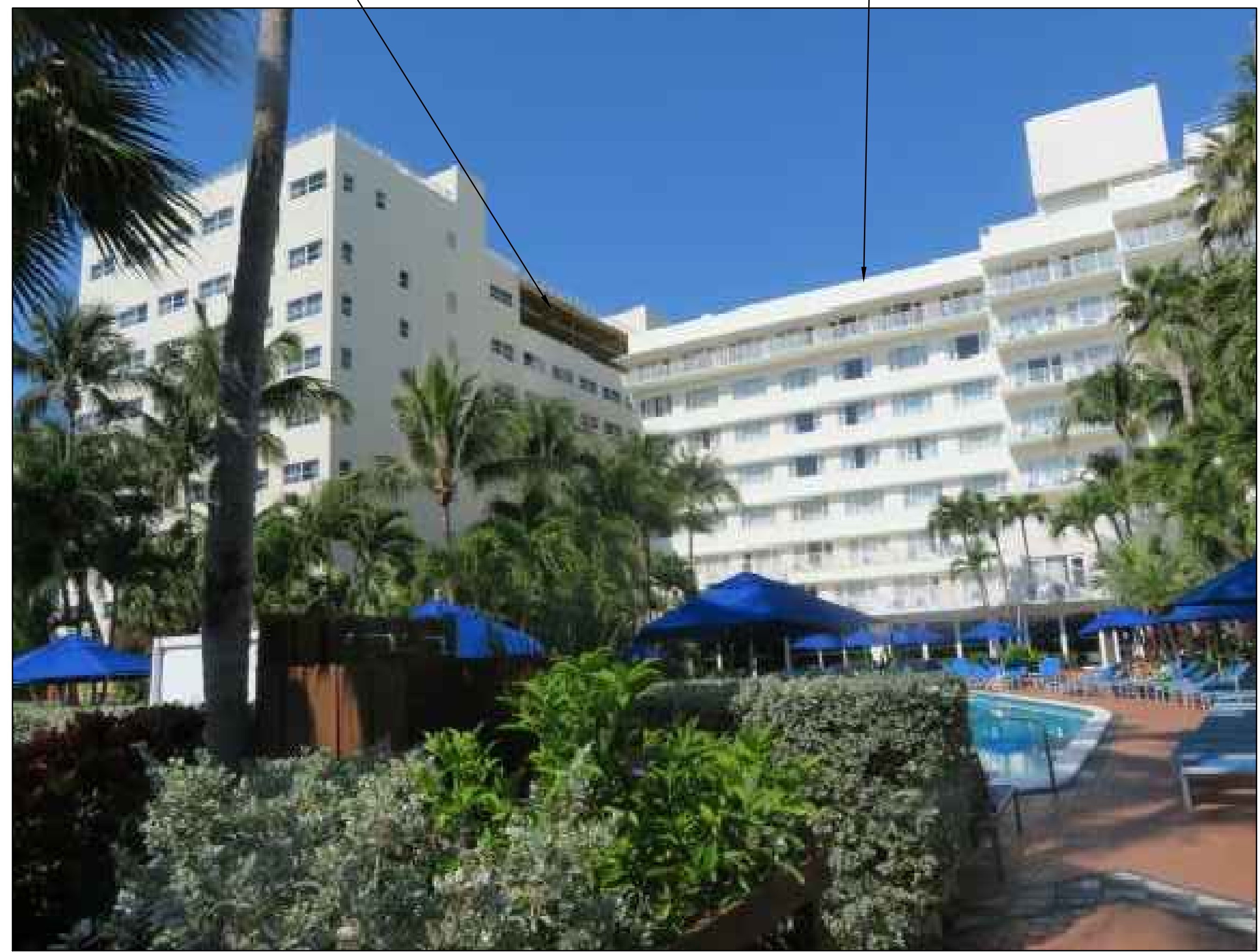
2 NORTH ELEVATION, VIEW FROM FOUR POINT HOTEL AREA IN SCOPE OF WORK, 11TH FLOOR SEE ARCHITECTURAL ELEVATION, SHEET A-4.1 PHOTO, DATED 4.3.2019
