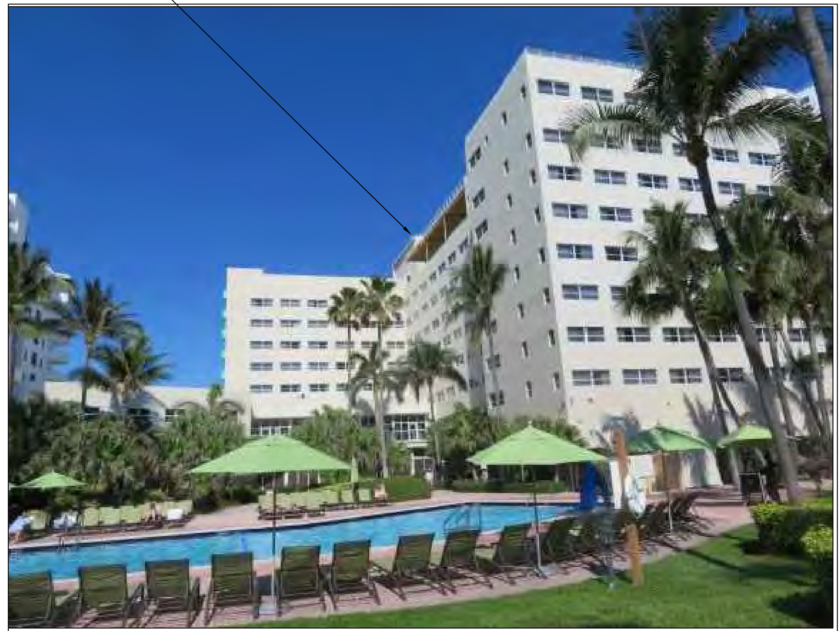
3 SOUTH ELEVATION, VIEW FROM THE POOL AREA IN SCOPE OF WORK, 11TH FLOOR SEE ARCHITECTURAL ELEVATION, SHEET A-4.2 PHOTO, DATED 4.3.2019
