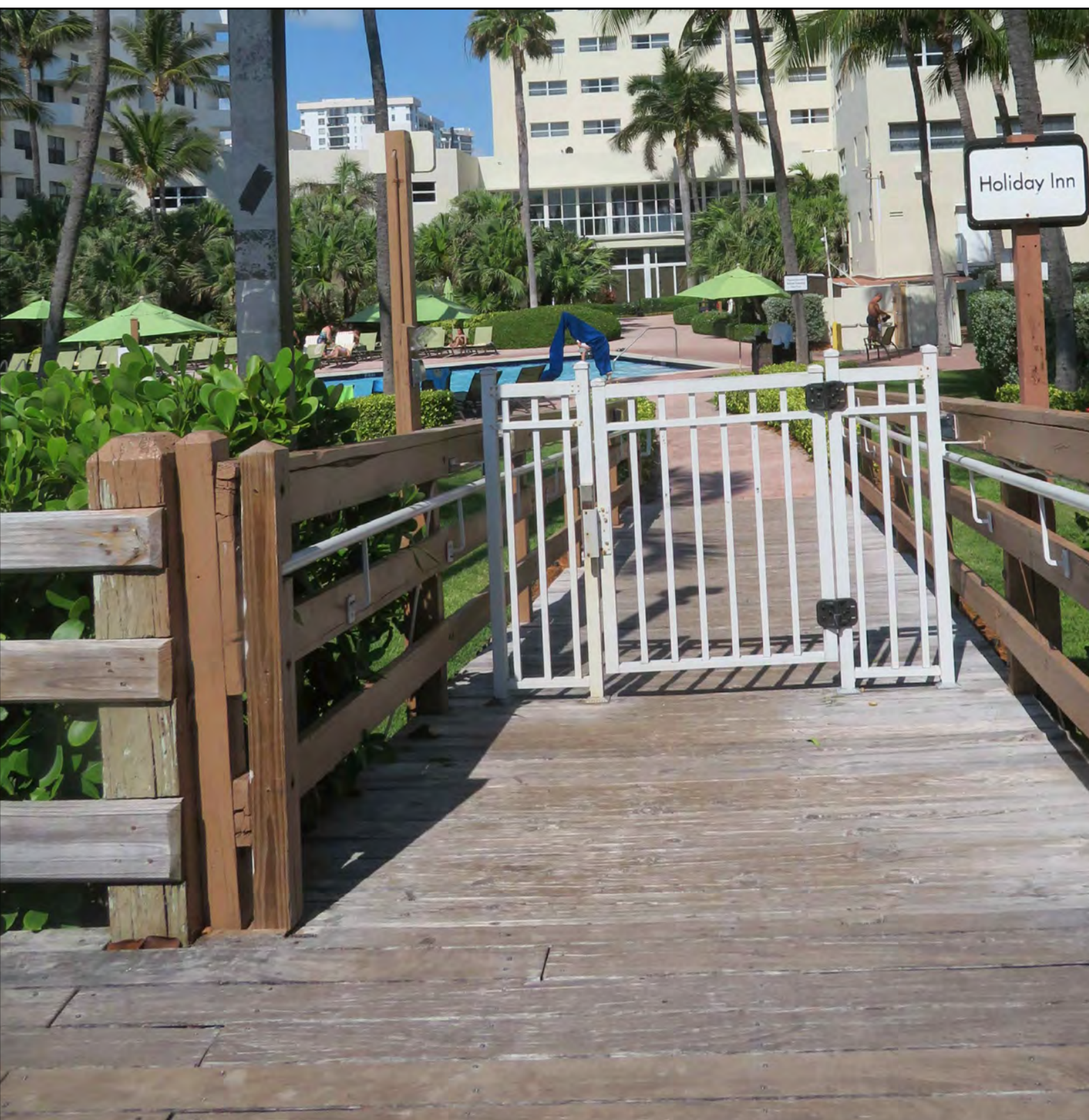
5 EAST ELEVATION, VIEW FROM THE BOARDWALK PHOTO, DATED 4.6.2019
