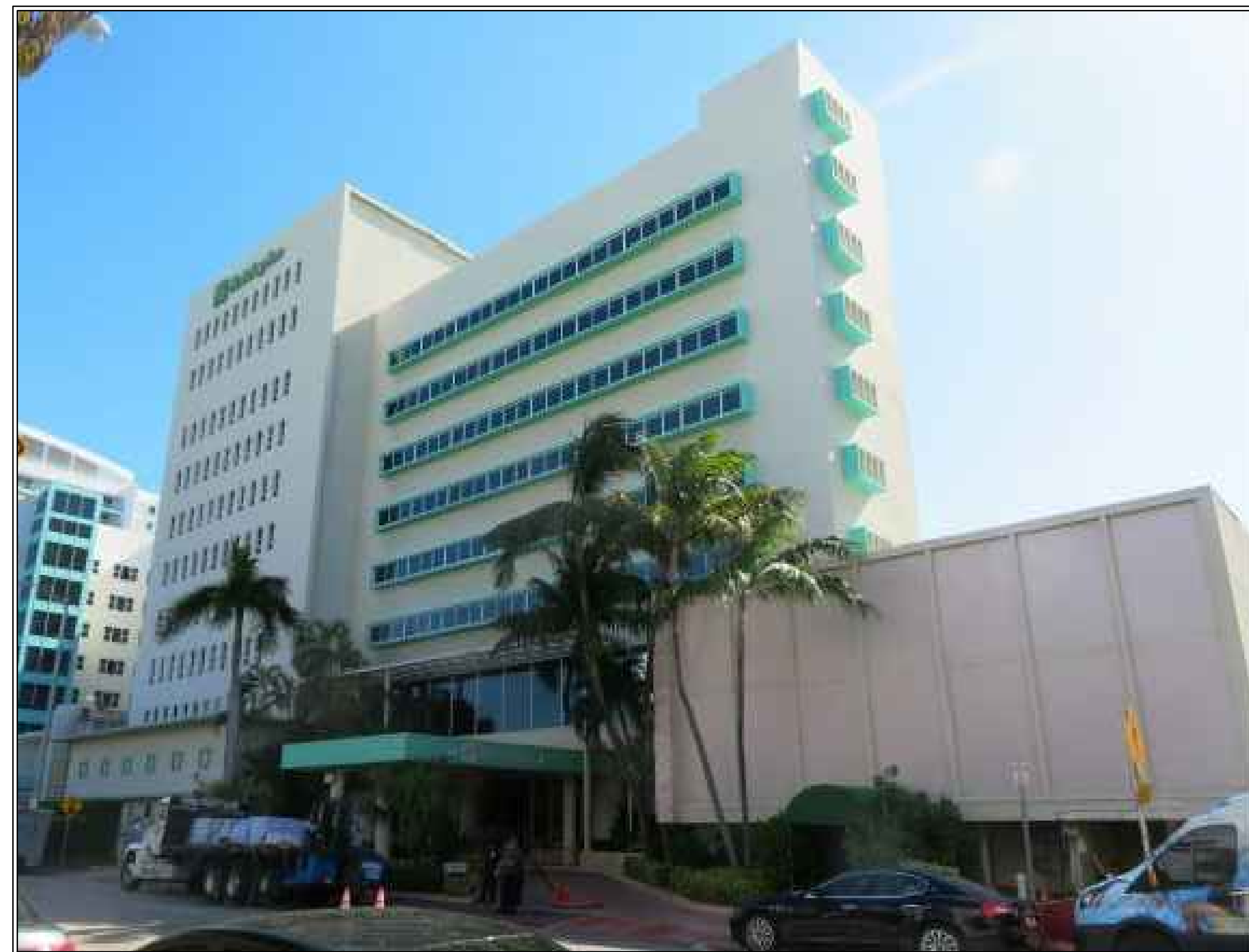
1 WEST ELEVATION, VIEW FROM COLLINS AVENUE NOT IN SCOPE OF WORK SEE ARCHITECTURAL ELEVATION, SHEET A-4.4 PHOTO, DATED 4.3.2019
