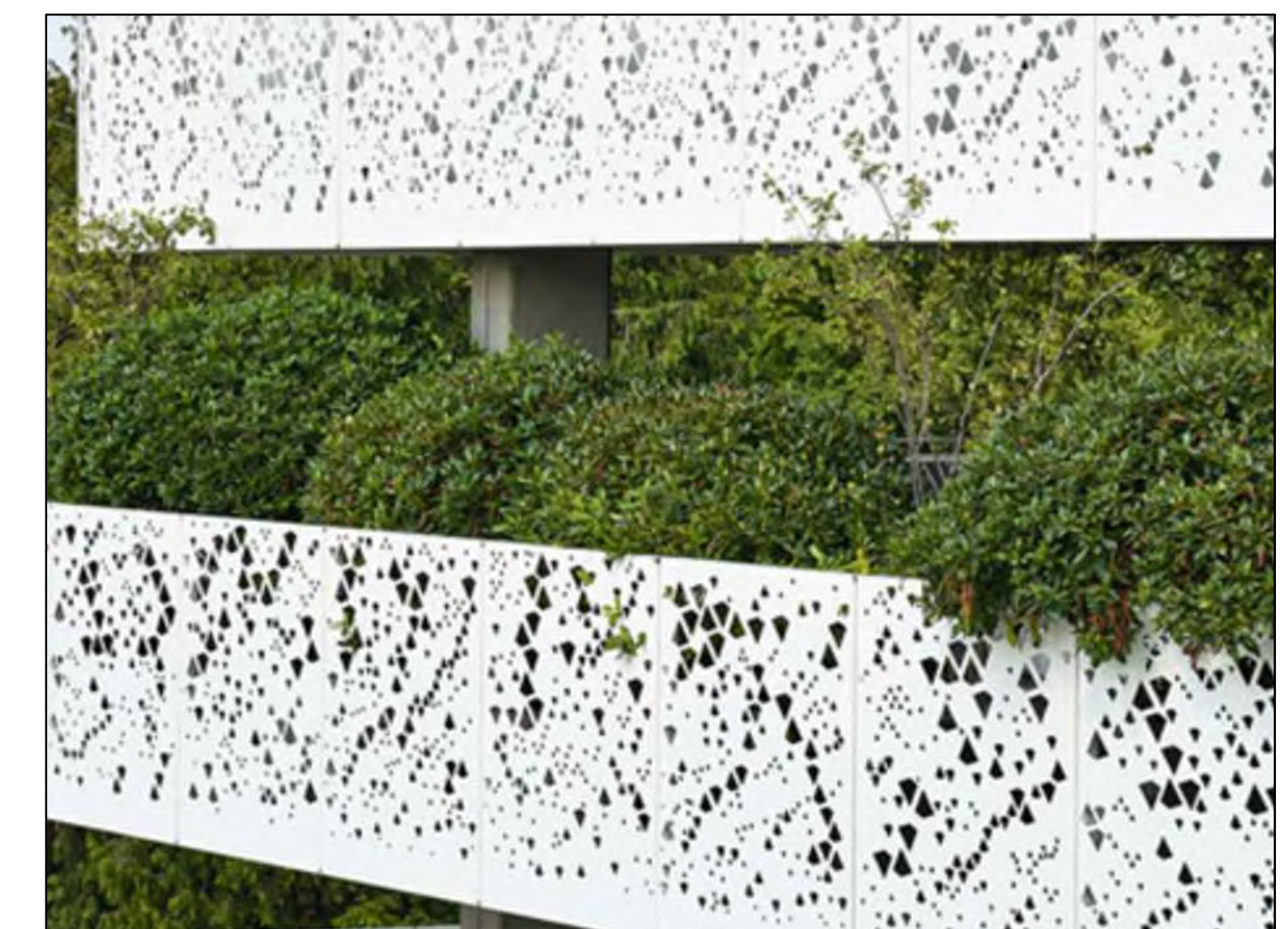
06 - PERFORATED METAL RAILING
